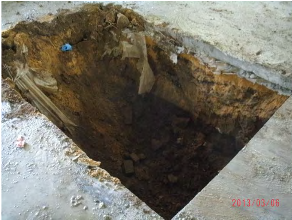
Photograph 3: Note urban fill consisting of bricks at start of excavation and that no hydraulic lift was observed.
