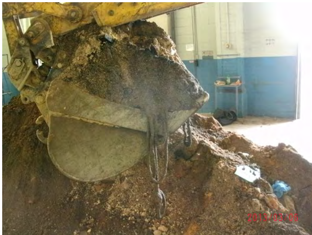
Photograph 4: Urban fill consisting of glass, rope and apparent ash as excavation is extended in depth.
