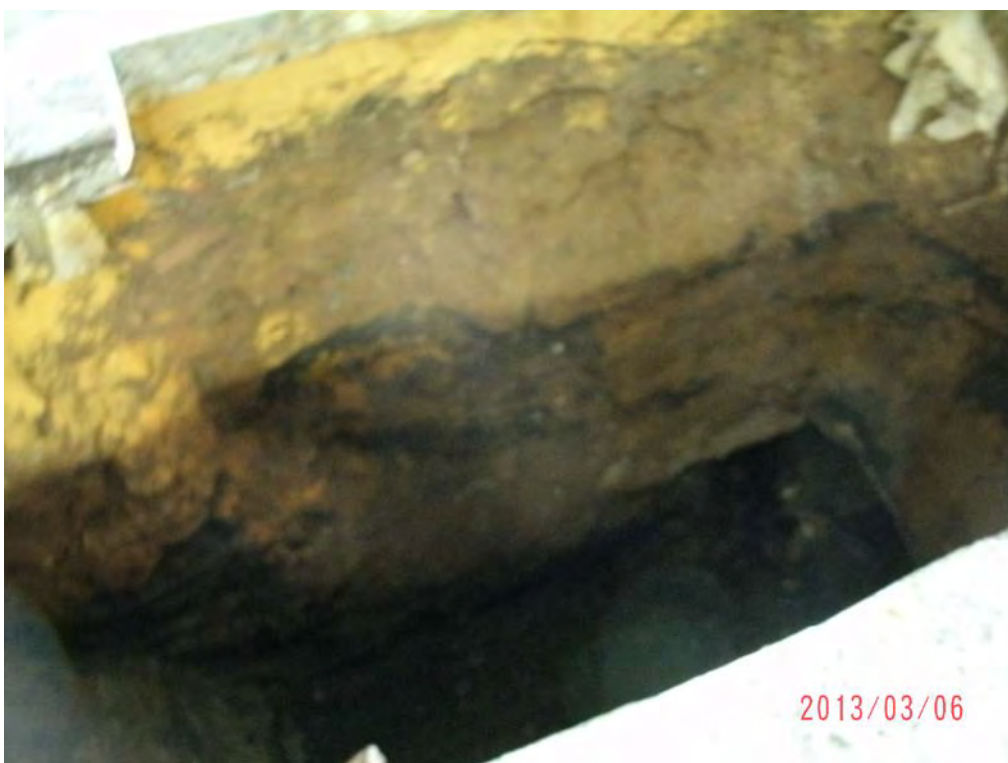
Photograph 6: Excavation extended in size to 11-feet below grade.
