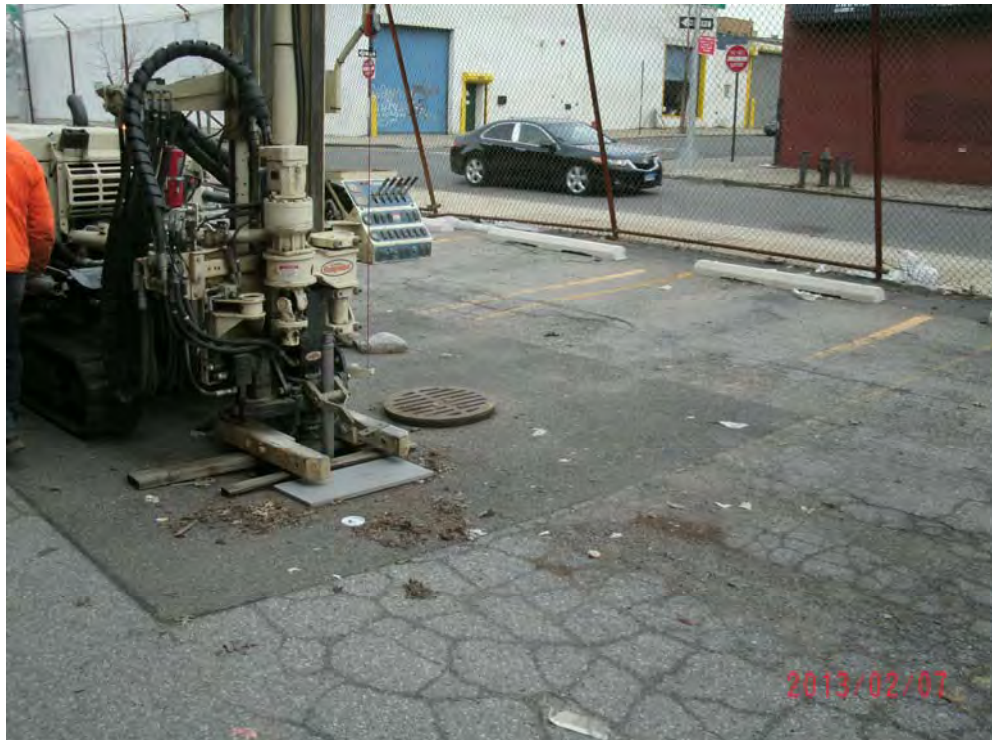
Photograph 13: Confirmatory boring in catch basin to determine structure has a solid concrete bottom.
