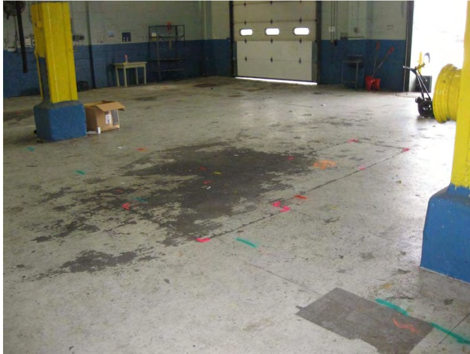
Photograph 5: Suspected concrete patch for former hydraulic lift
