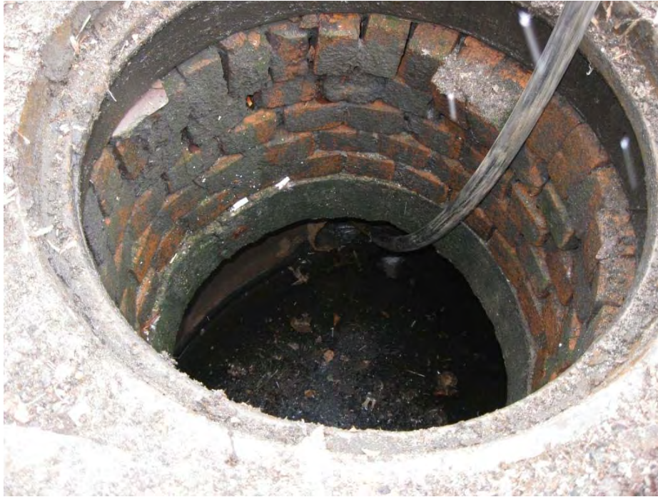
Photograph 7: Catch basin with drainage pipe
