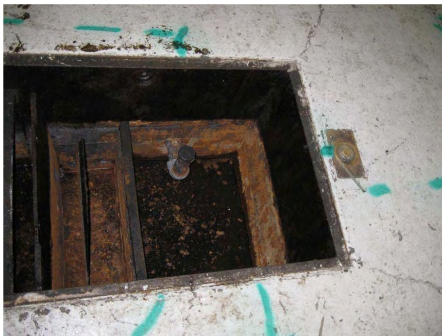
Photograph 2: Oil/water separator vault with capped line
