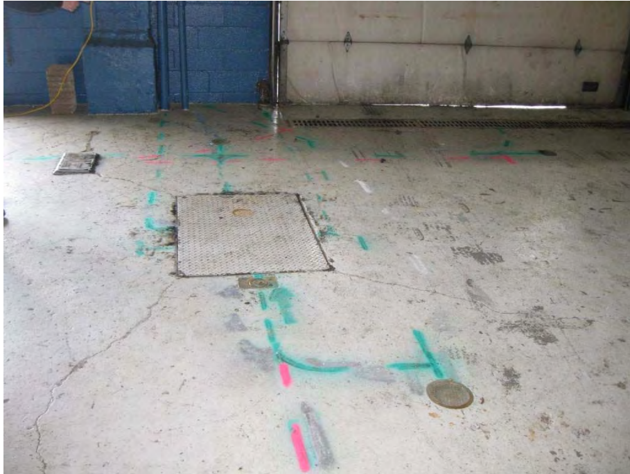
Photograph 3: Drainage lines for oil/water separator
