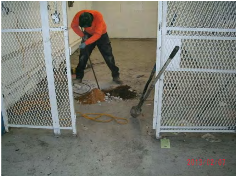
Photograph 13: Installation of GP-7 proximate to waste oil UST within caged area of garage.
