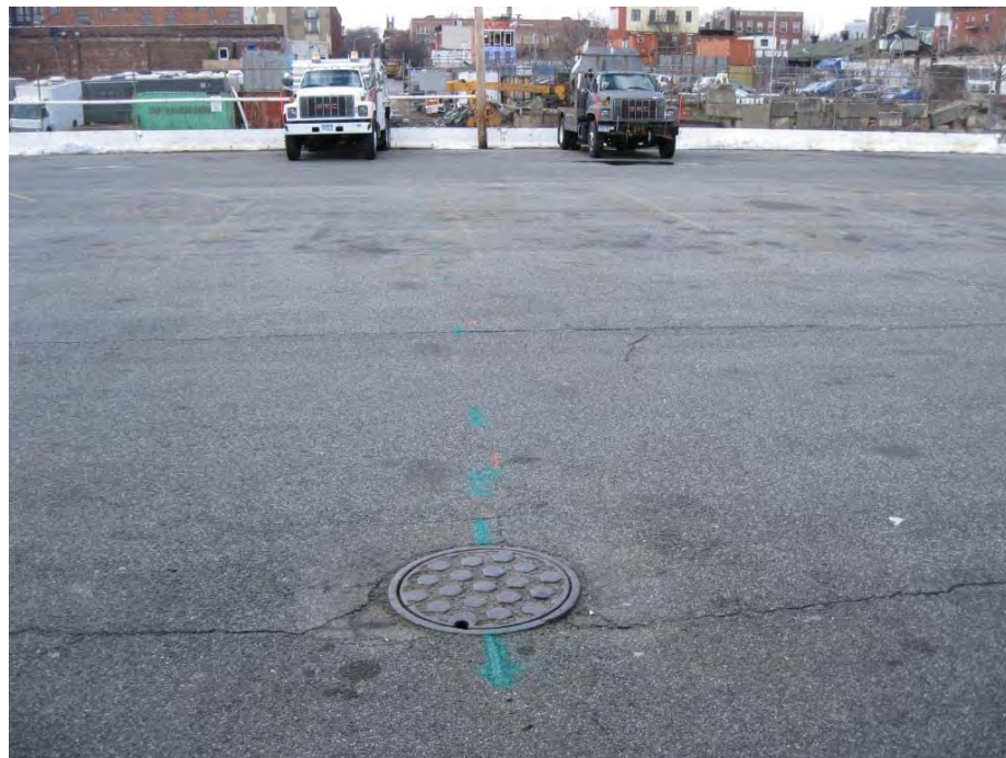
Photograph 6: Building's rear sanity sewer line
