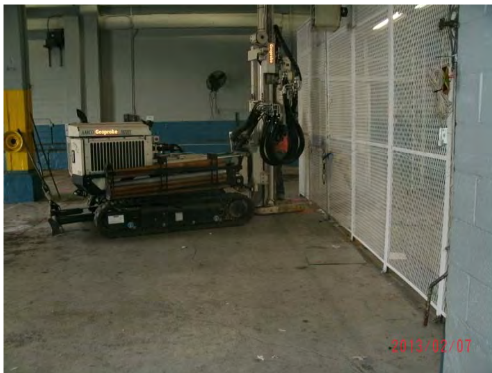
Photograph 11: Installation of GP-6 proximate to waste oil UST.
