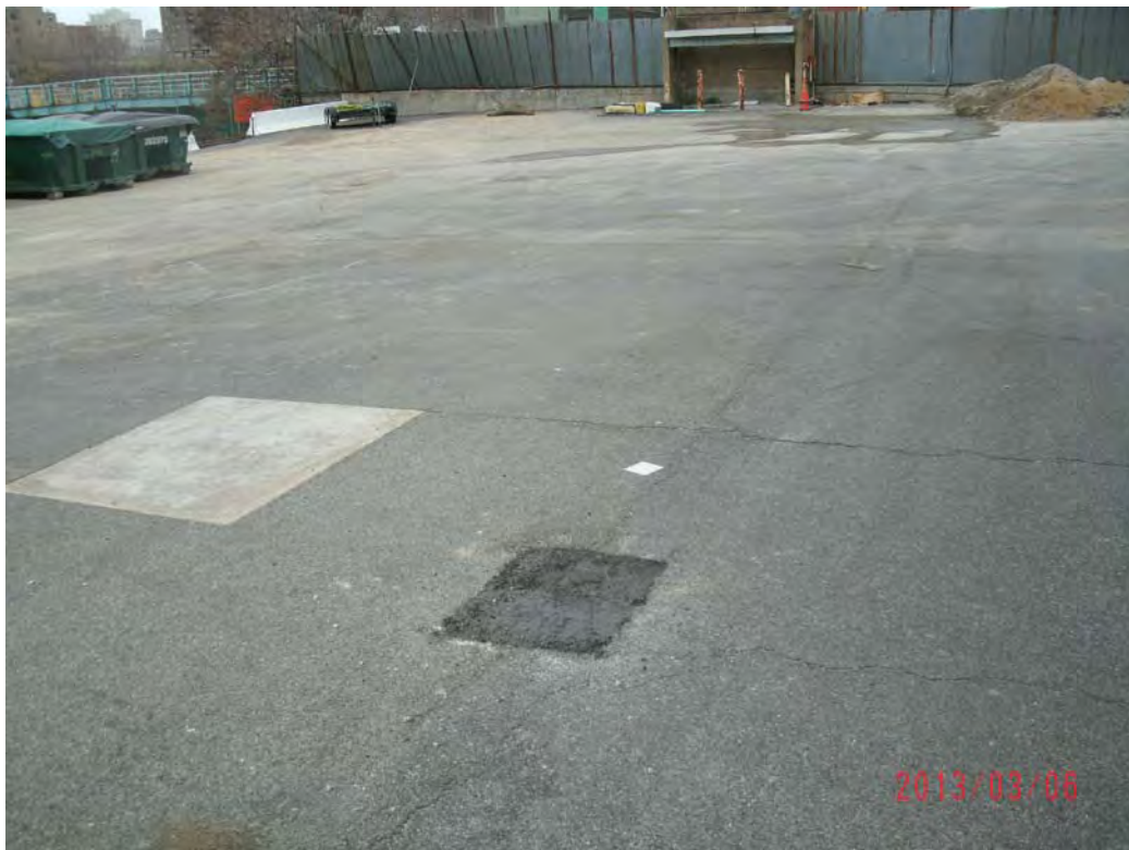
Photograph 10: Completed abandonment of on-site monitoring well.
