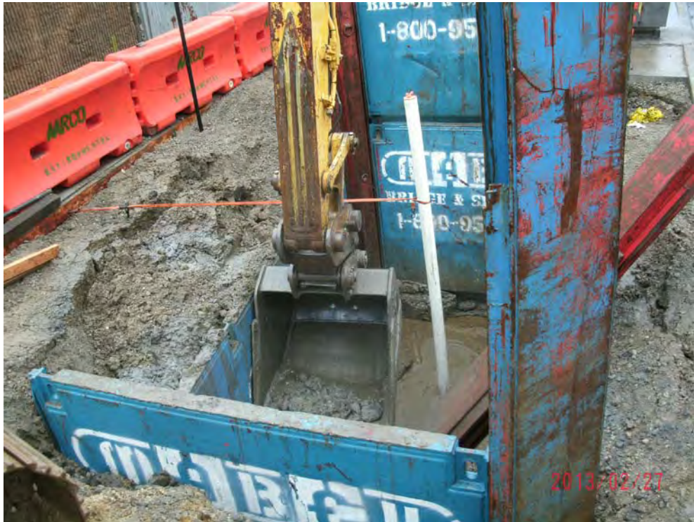
Photograph 7: Excavation of 2 nd half of sidewalk and installation of replacement well #8.
