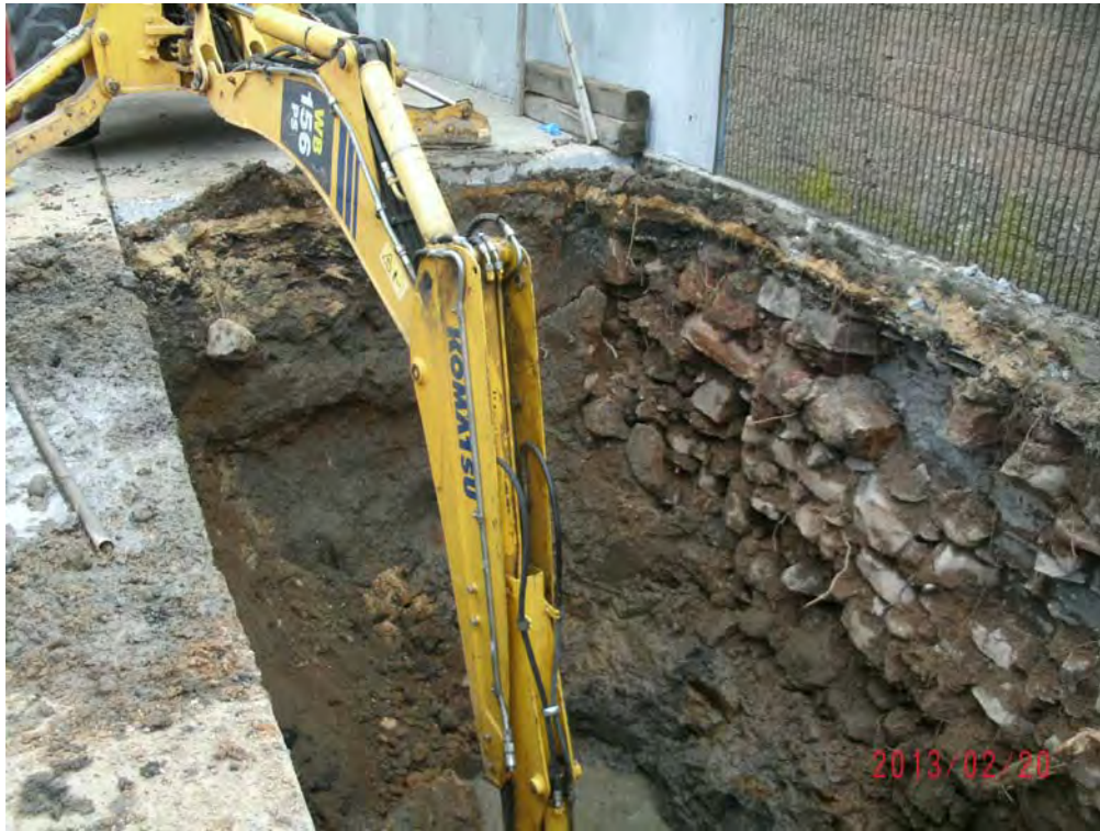
Photograph 3: 1st half of sidewalk excavation. Note rock retaining wall at southern sidewall.
