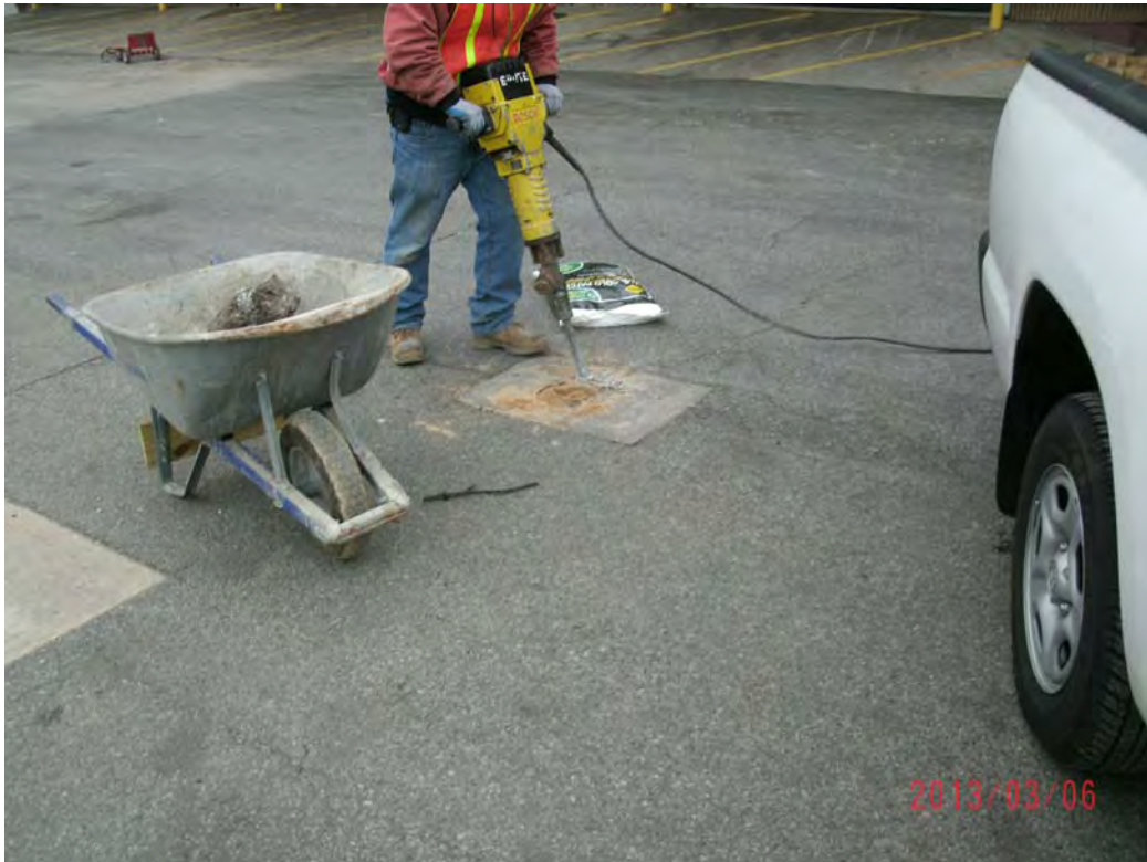
Photograph 9: Abandonment of on-site monitoring wells.
