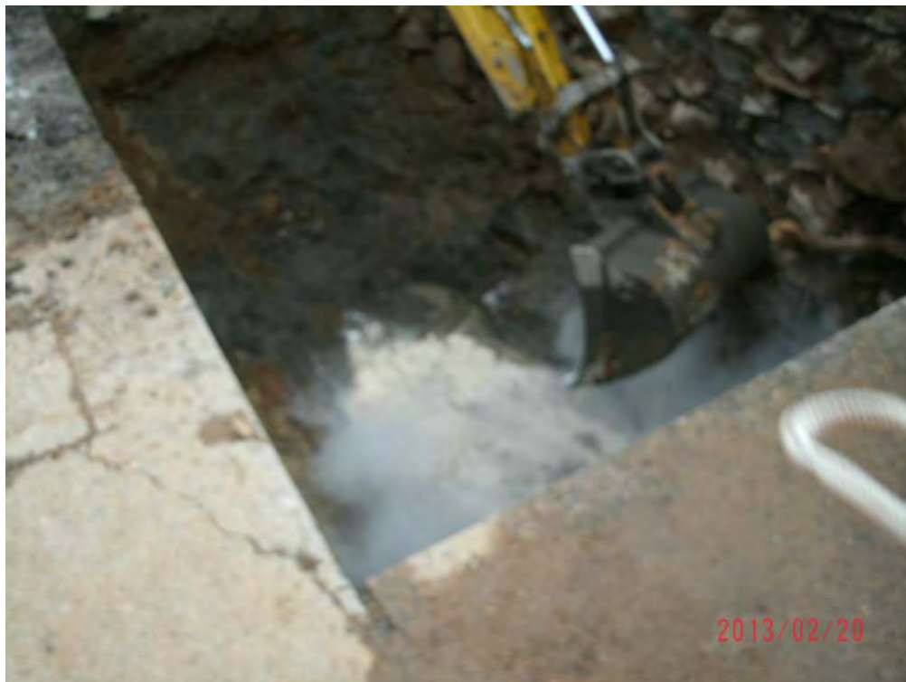
Photograph 4: Application of RegenOx and ORCA to excavation.
