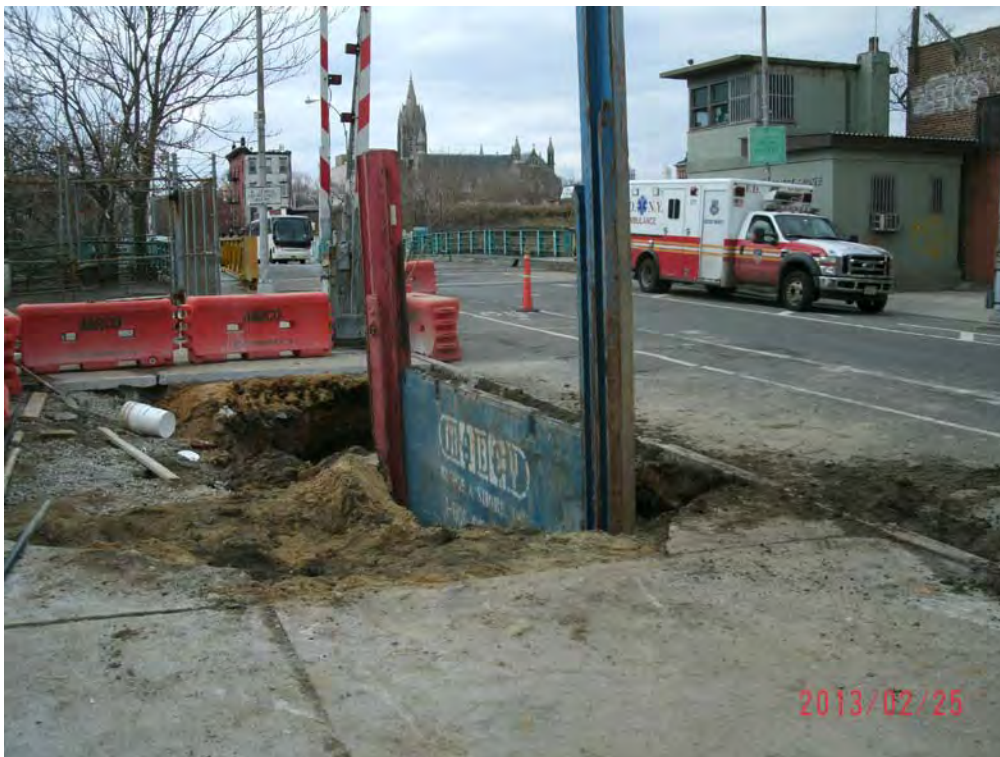
Photograph 6: Installation of shoring for road stabilization.
