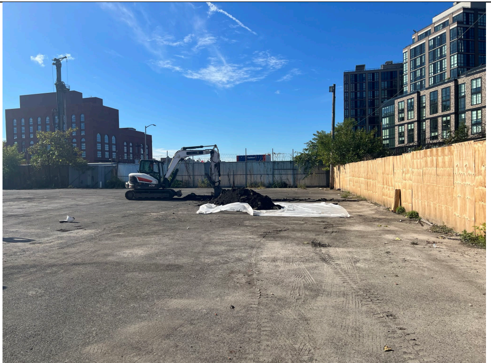
Photo 2 – Representative photo of Xolle placing material from test pit on poly sheeting.
