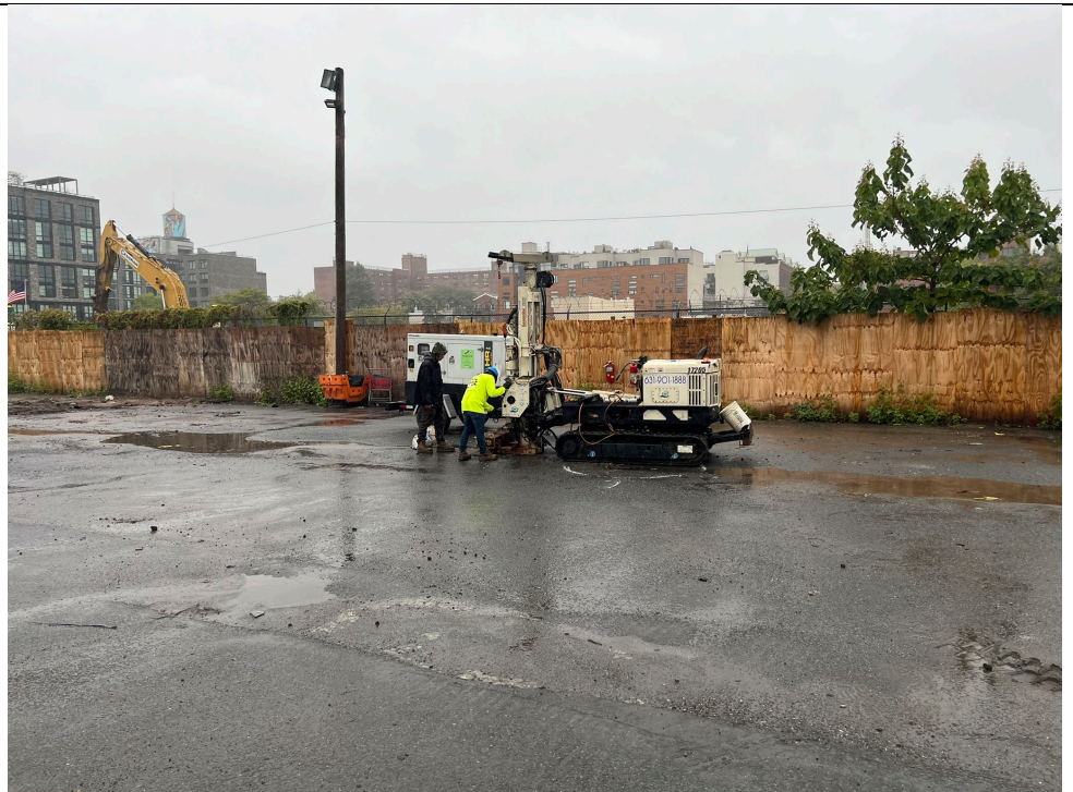
Photo 2 – Representative photo of drilling SV-4.
