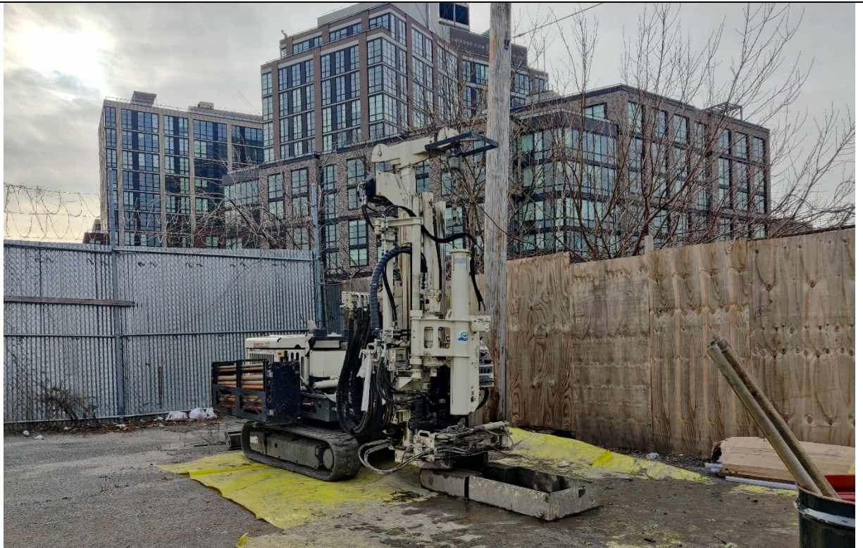
Photo 4- View of the 20' step off location to SB-16-S1, to the south, designated as SB-16-S2. Step off boring location which will begin installation on 11/12/23.
