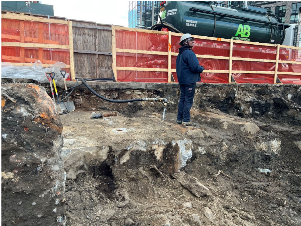
Photo 2 – Representative photo of AB environmental pumping water out of tanks
