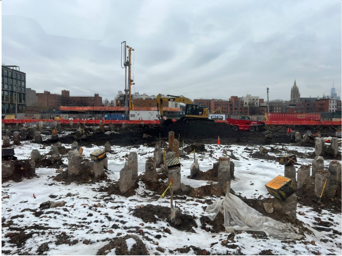
Photo 5 – Representative photo of excavation on the southern portion of the Site.
