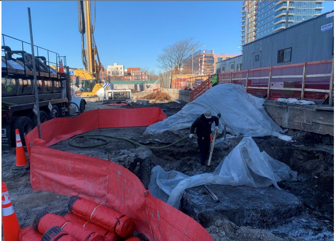
Photo 4 – Representative photo of PAL pumping out Tank-11.
