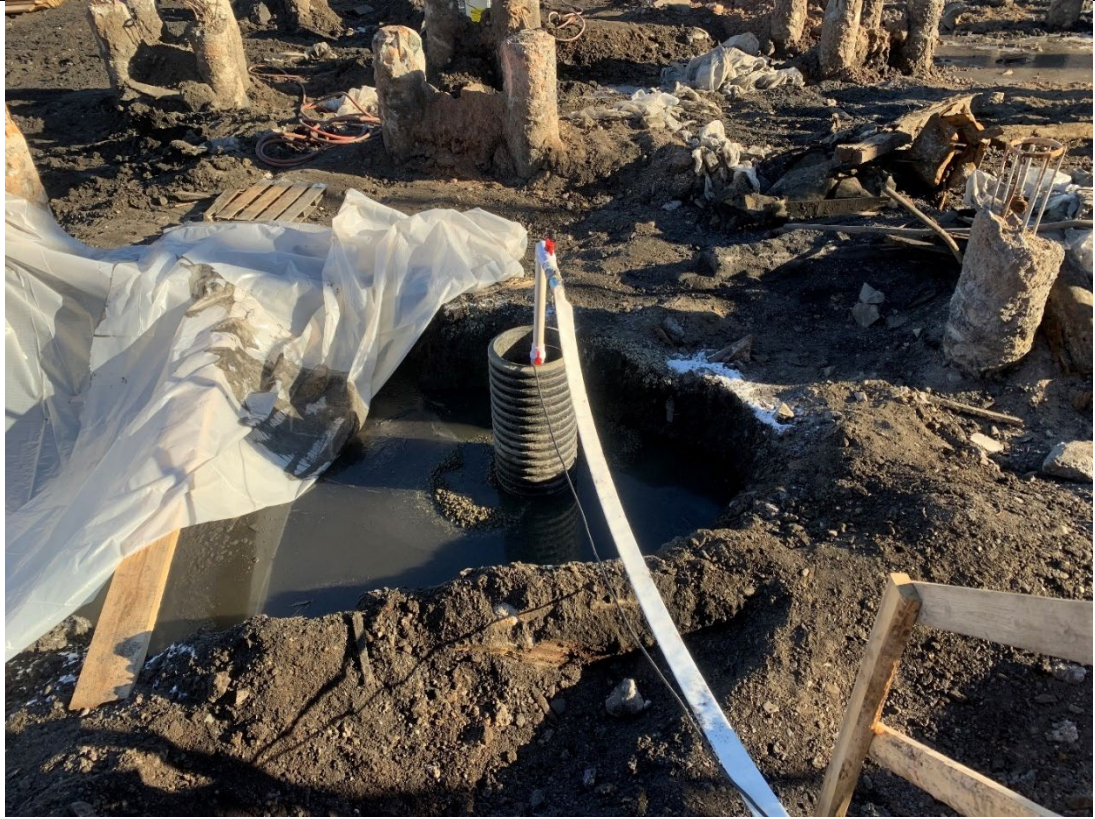
Photo 3 – Representative photo of dewatering in grid A5.
