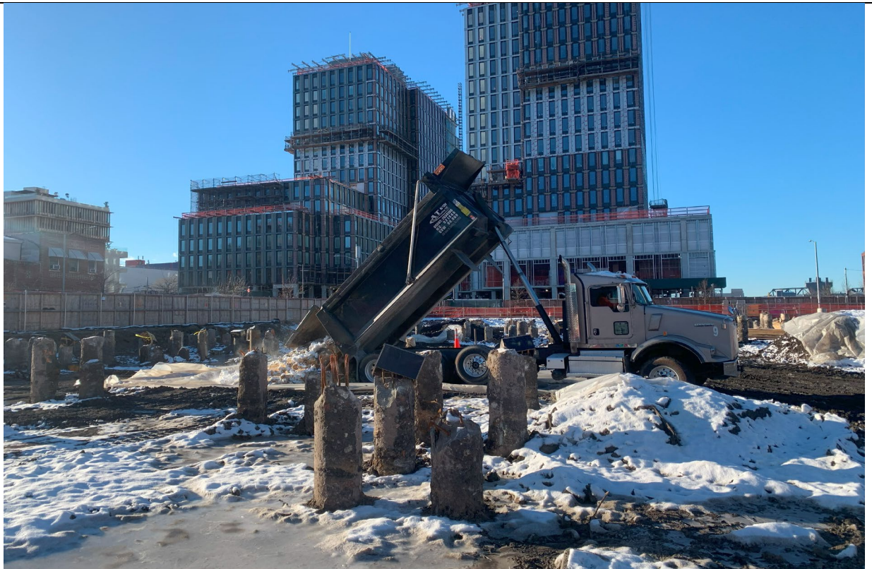
Photo 2 – Representative photo of approved crushed limestone being unloaded on grid E6.
