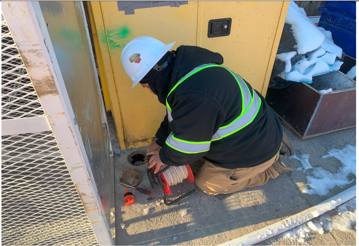
Photo 1 – Representative photo of dewatering well gauging.
