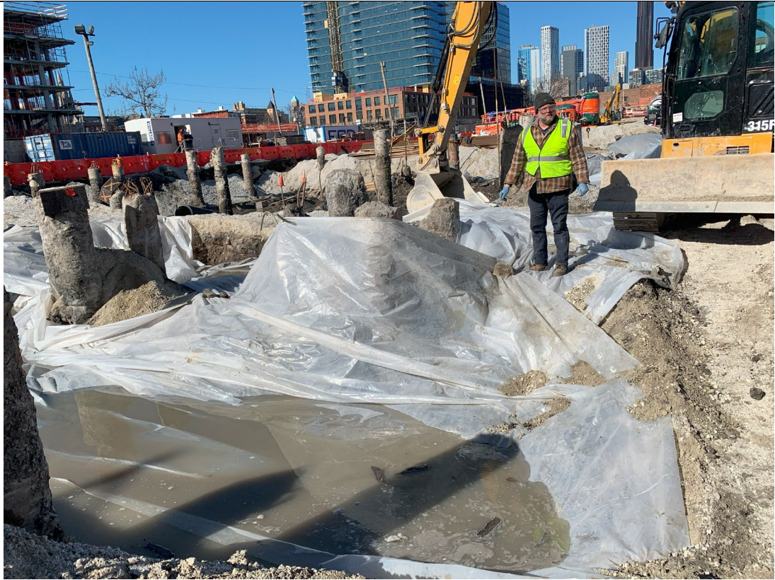
Photo 1 – Representative photo of poly sheeting coverage in grid B4.
