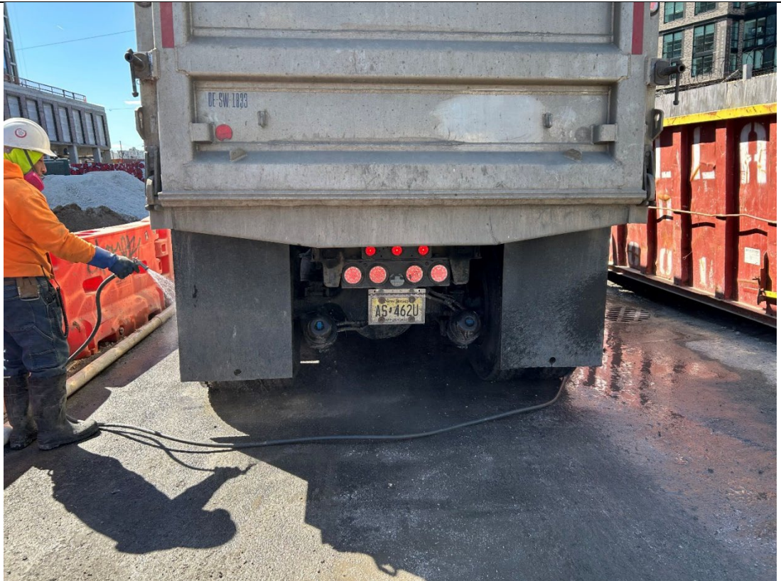
Photo 4 – Representative photo of tire washing over track pad.
