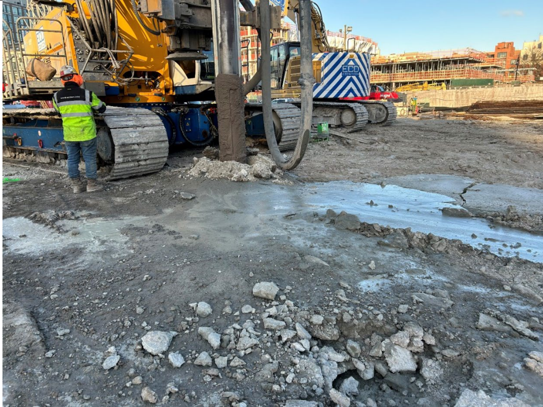
Photo 5 – Representative photo of pile installation in grid N5.
