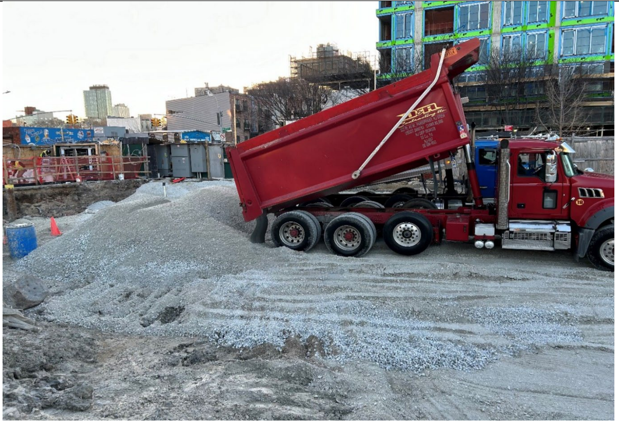
Photo 1 – Representative photo of imported fill being stockpiled in grid M6.
