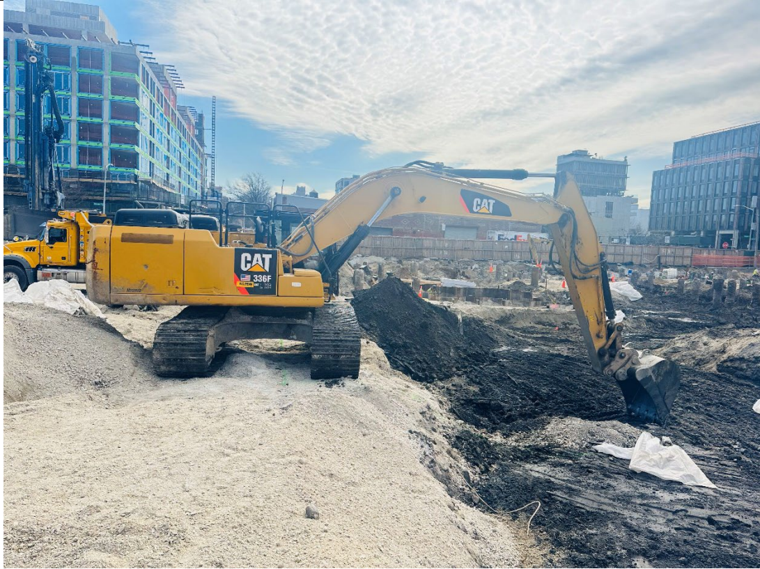
Photo 3 – Representative photo of soil excavation.
