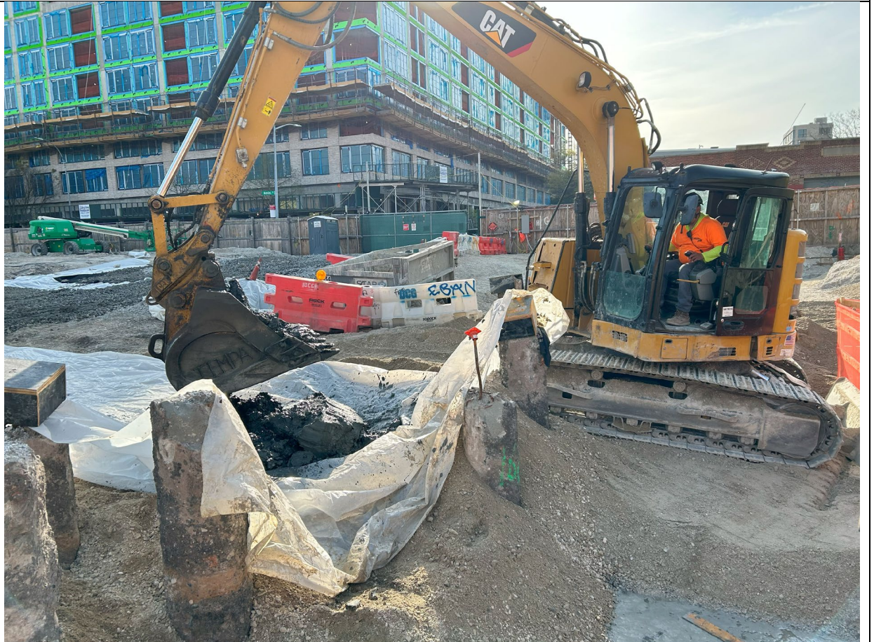
Photo 4 – Representative photo of SB-13 excavation.
