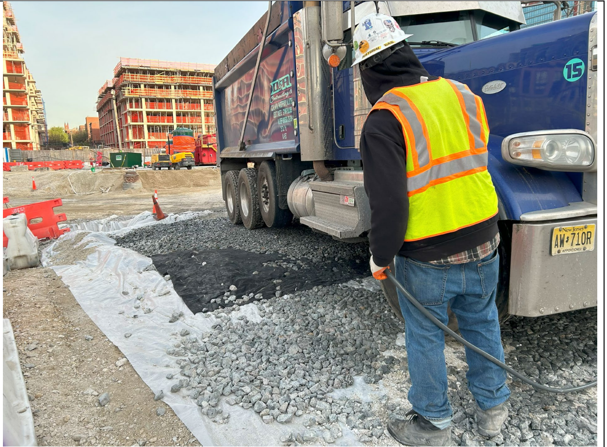
Photo 3 – Representative photo of tire washing over temporary track pad.
