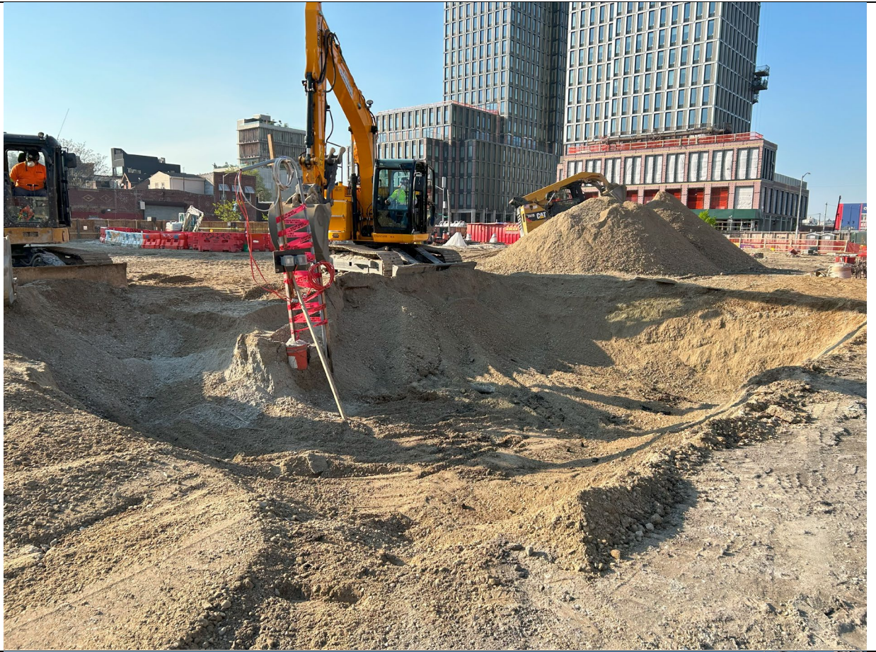
Photo 1 – Representative photo of excavation of grid H2.
