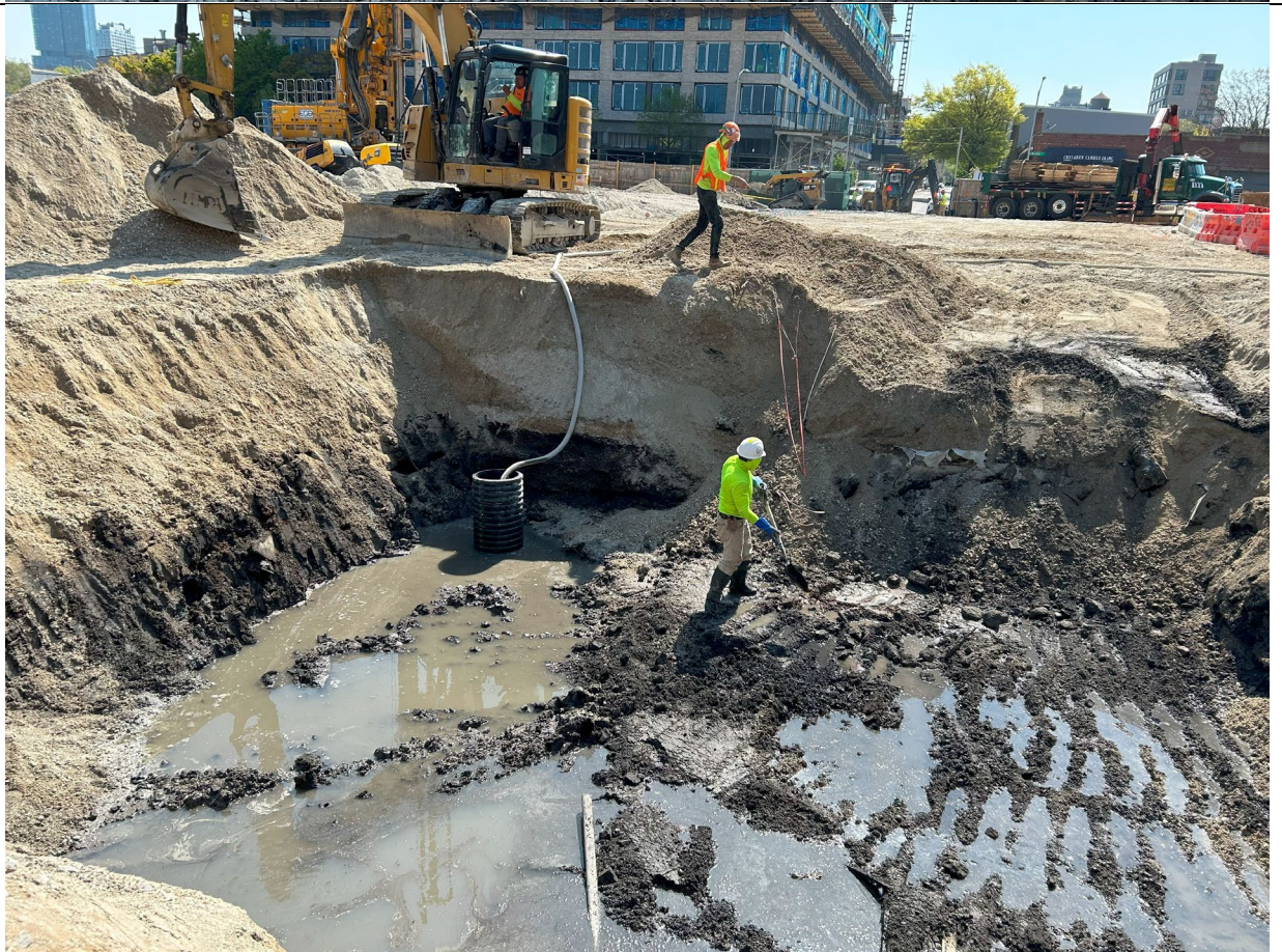
Photo 4 – Representative photo of dewatering sump active in H2 excavation.
