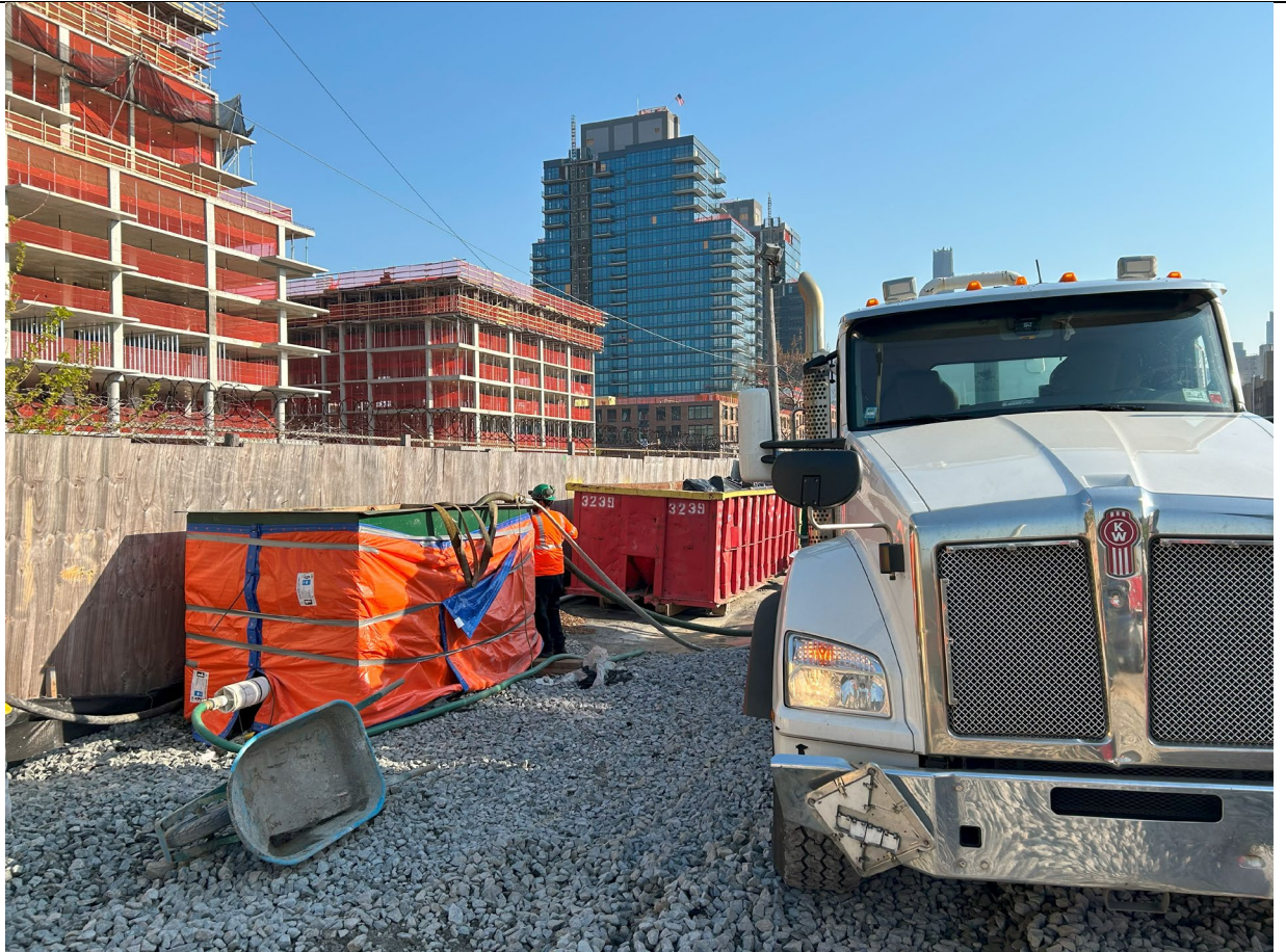
Photo 3 – Representative photo of Triumvirate pumping out Truck Wash Frac Tank.
