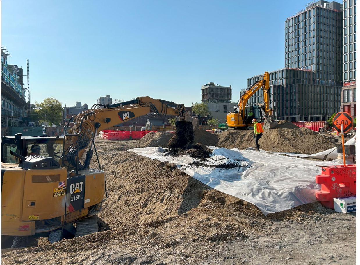
Photo 2 – Representative photo of soil stockpile from grid H2 being placed on top of poly sheeting.
