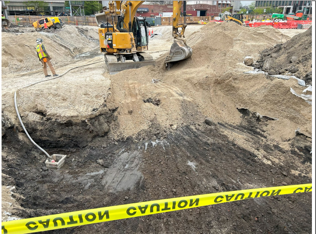
Photo 1 – Representative photo of excavation of grid J2.
