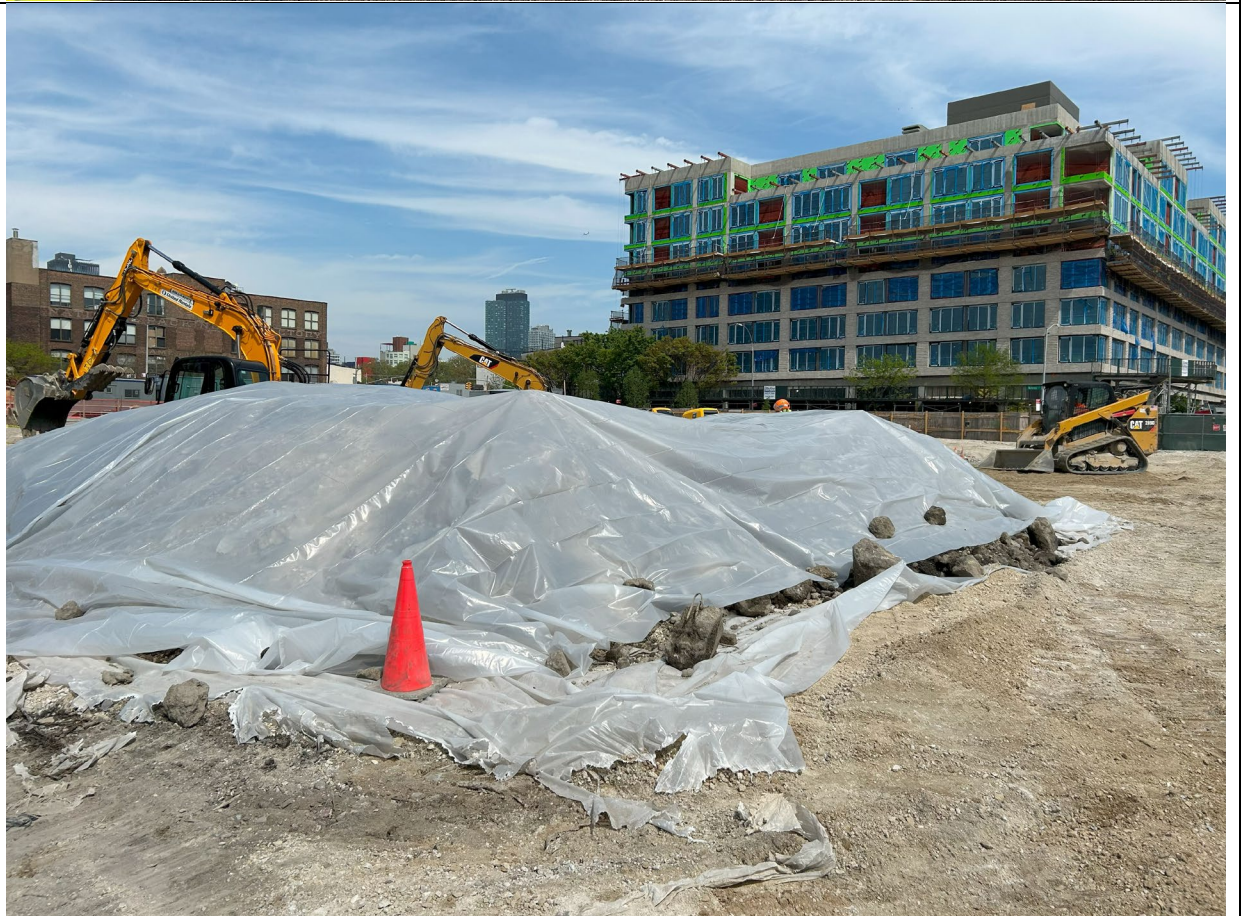
Photo 2 – Representative photo of soil stockpile covered with poly sheeting.
