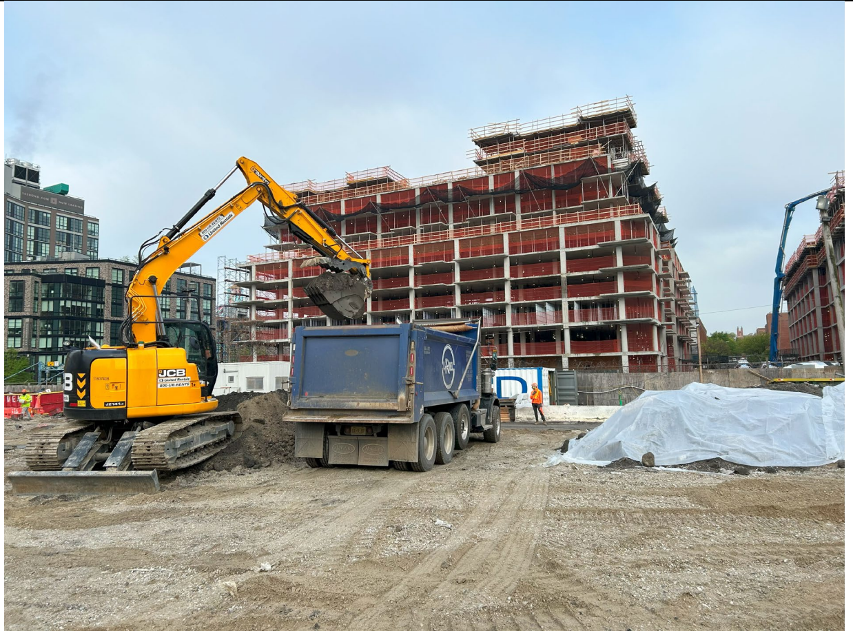
Photo 1 – Representative photo of material load out.
