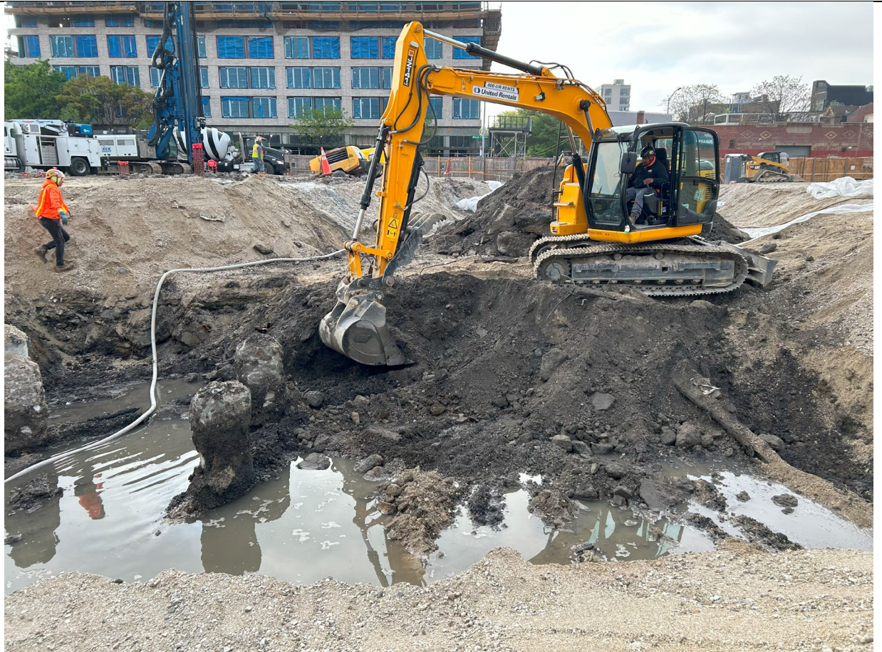
Photo 5 – Representative photo of Excavation in grid J3.
