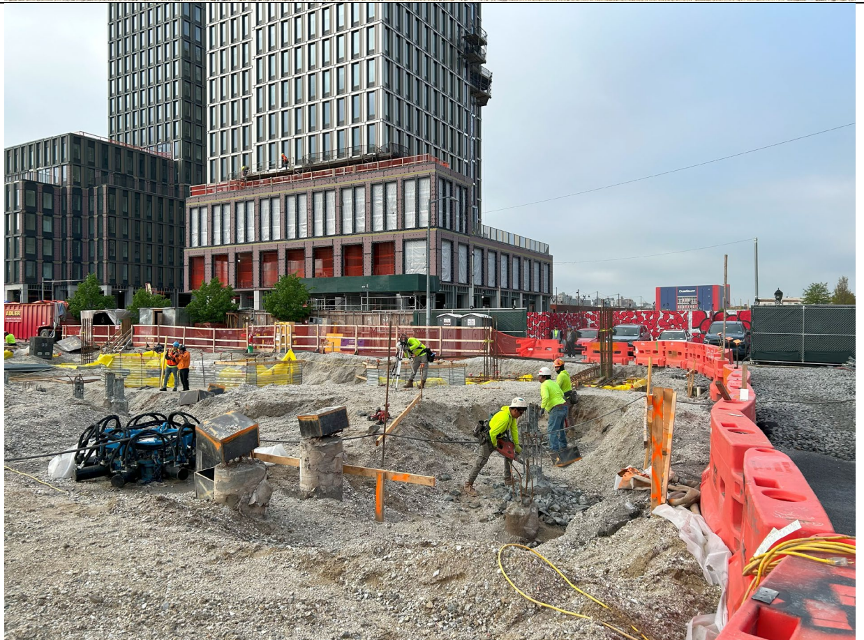
Photo 6 – Representative photo of pile cap work in grid B2.
