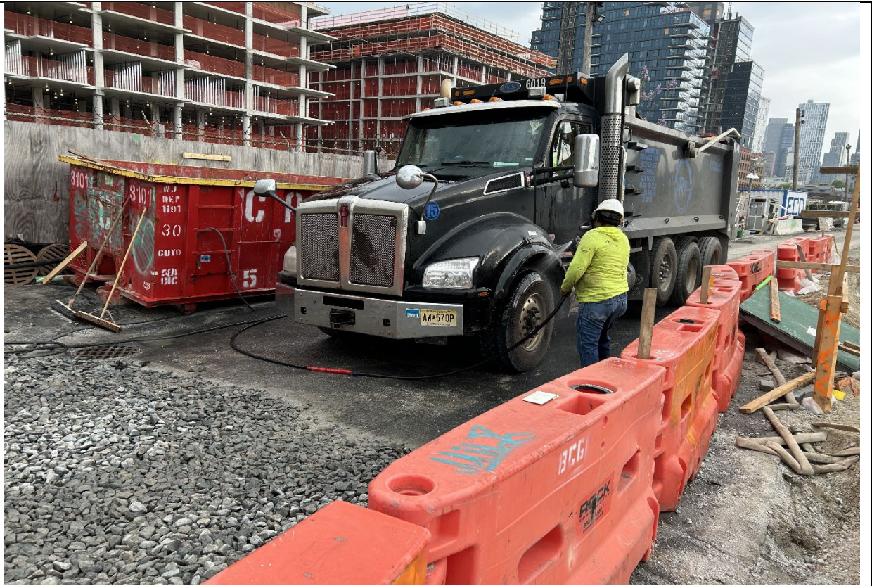
Photo 1 – Representative photo of truck tires being washed over track pad.
