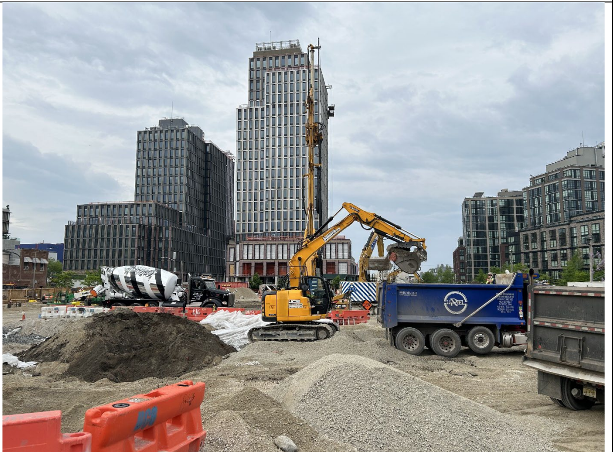
Photo 2 – Representative photo of soil load out.
