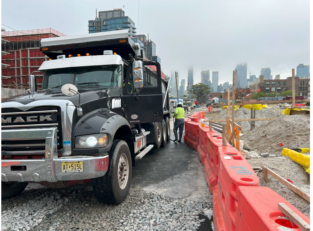
Photo 1 – Representative photo of truck- wash station.
