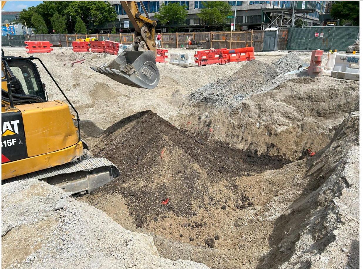
Photo 2 – Representative photo of excavation of grid H5.
