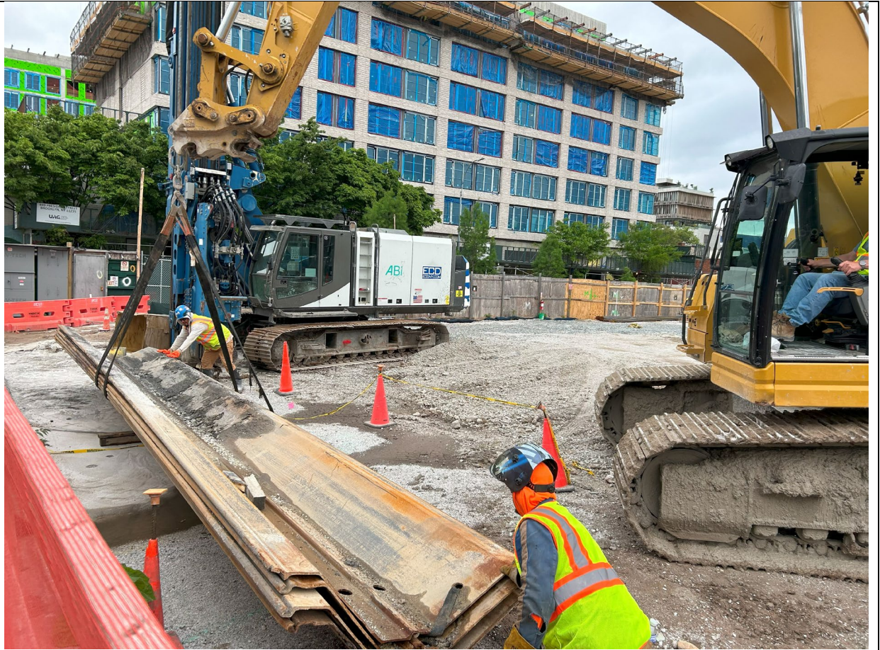
Photo 3 – Representative photo of sheet pile staging on grid O7.
