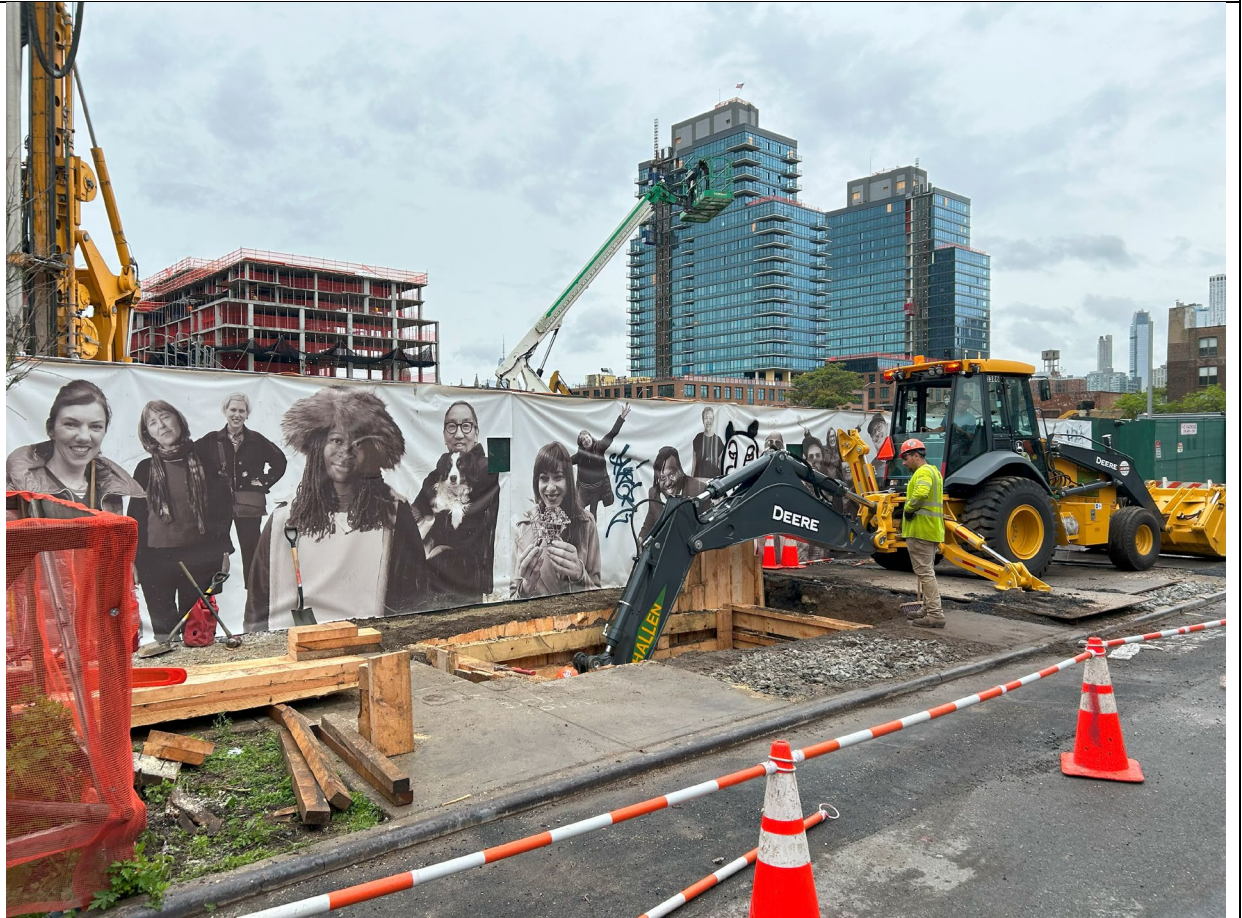
Photo 4 – Representative photo of National grid trench excavation along Nevins Street.
