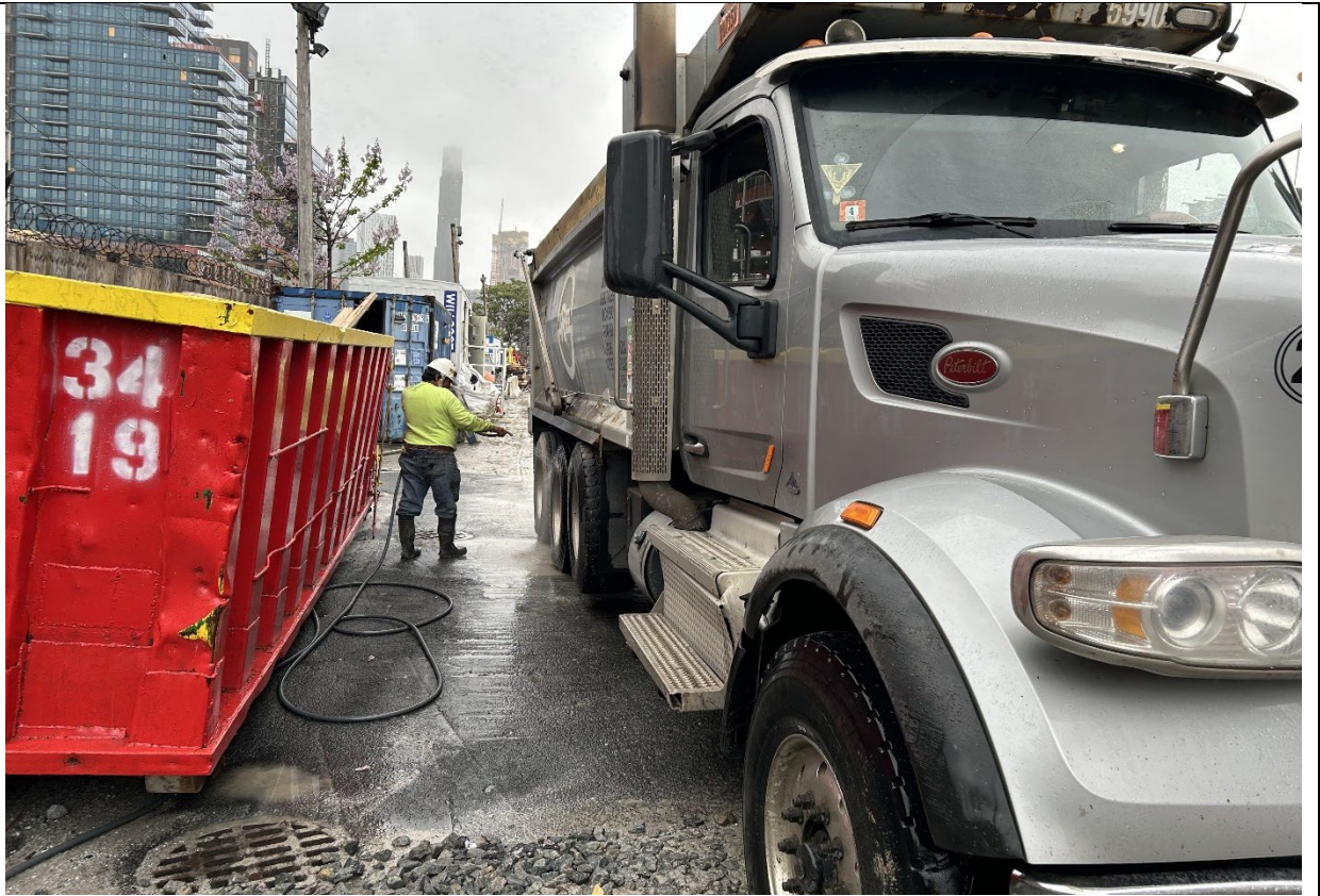
Photo 1 – Representative photo of truck- wash station over track pad
