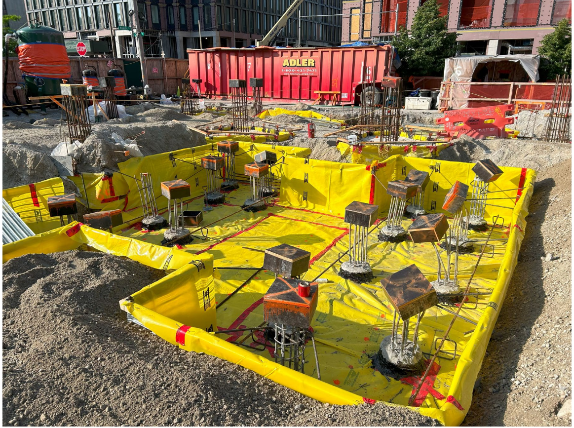
Photo 1 – Representative photo of vapor barrier and footing construction.
