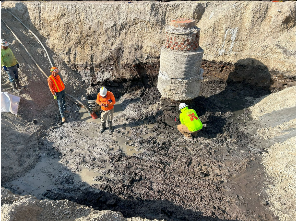
Photo 2 – Representative photo of excavated grid H4 and dewatering sump.
