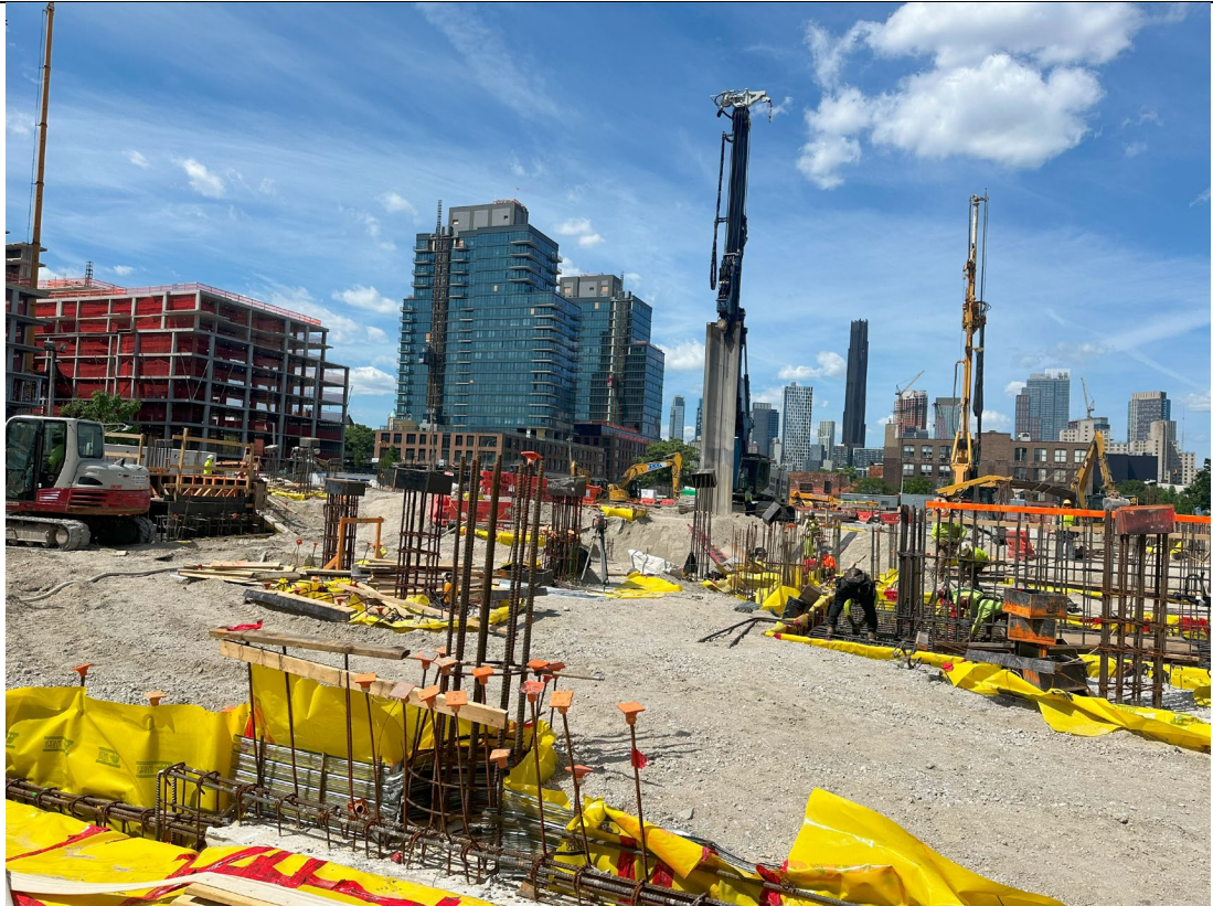
Photo 5 – Representative photo of KFS working on footing installation.
