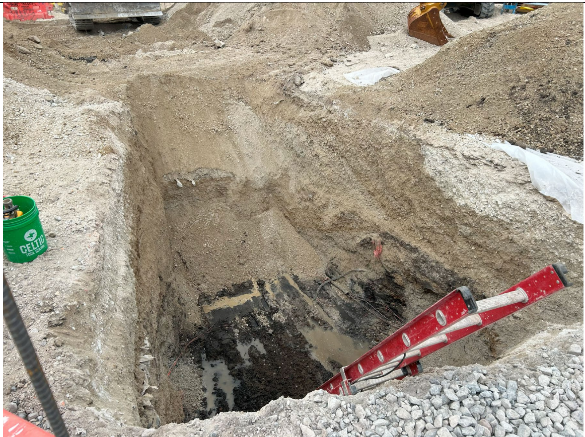
Photo 4 – Representative photo of SB-14 excavation.
