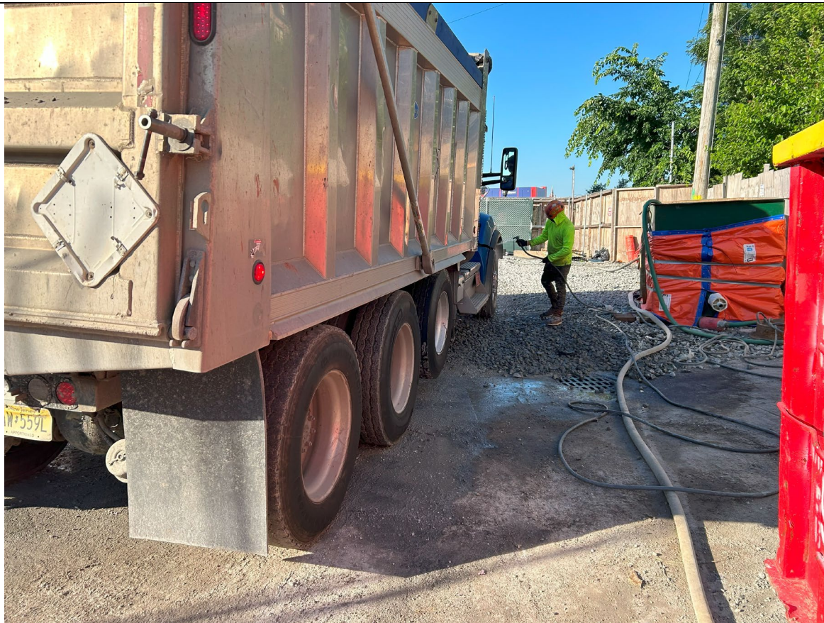
Photo 2 – Representative photo of tire washing over track pad.
