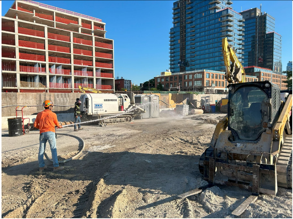
Photo 1 – Representative photo of dust suppression of truck roadway.
