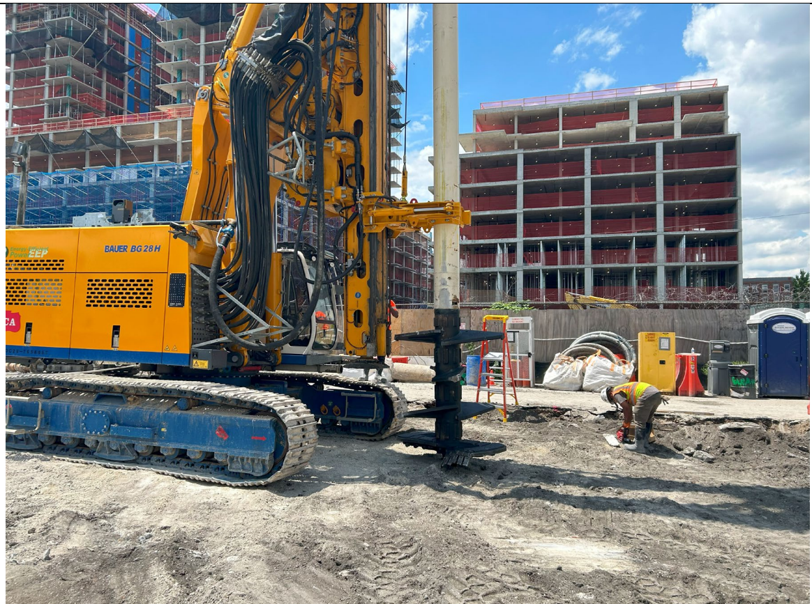
Photo 6 – Representative photo of 6' auger attached to ISS rig.
