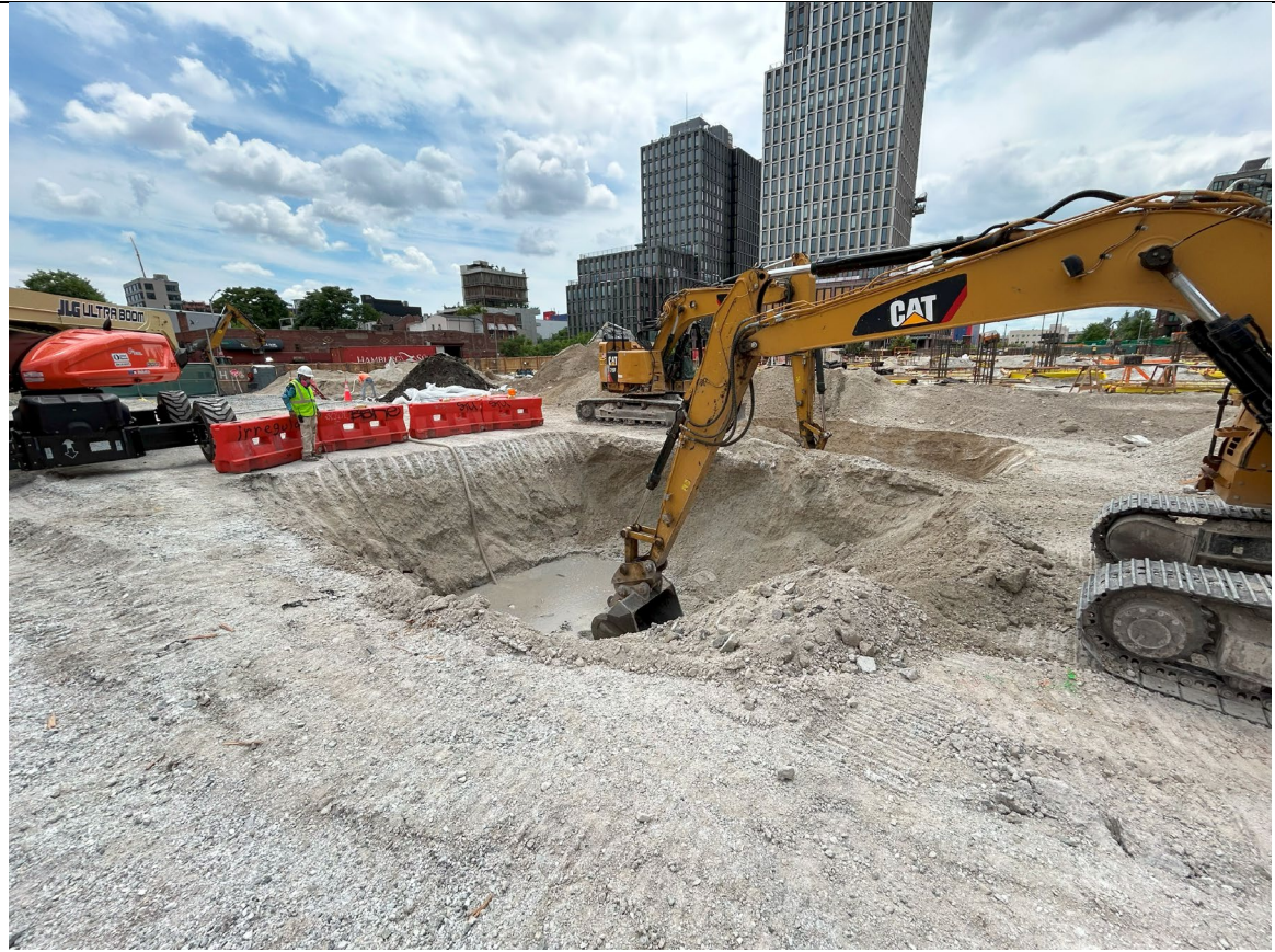
Photo 5 – Representative photo of EP-38 excavation.
