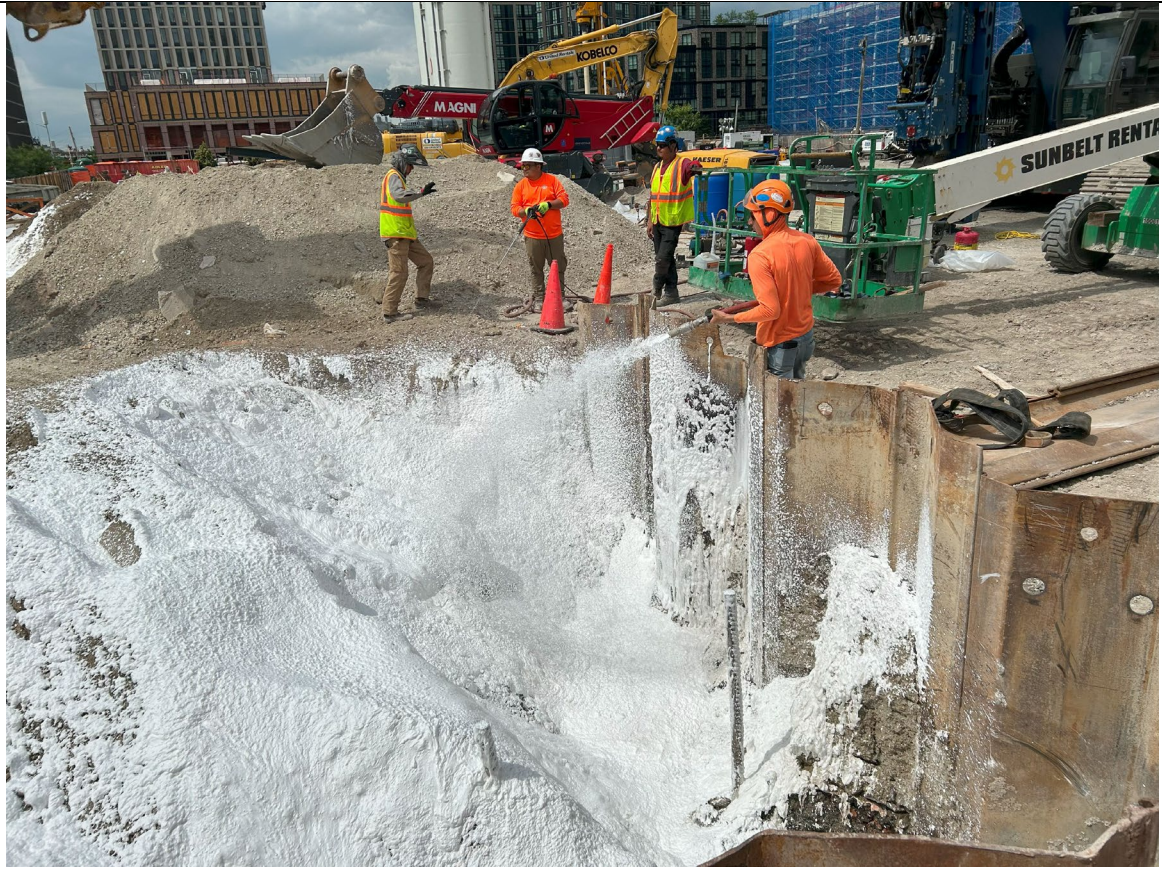
Photo 3 – Representative photo of preemptive odor suppression of Spill 2308807 area via ATMOS foam and Hydro Carbon Spray.
