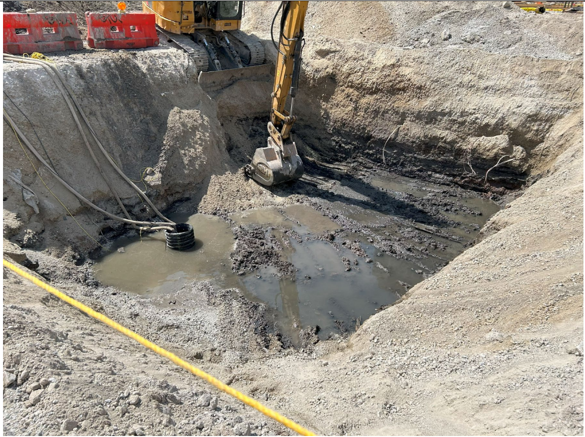
Photo 3 – Representative photo of dewatering active in grid H3.
