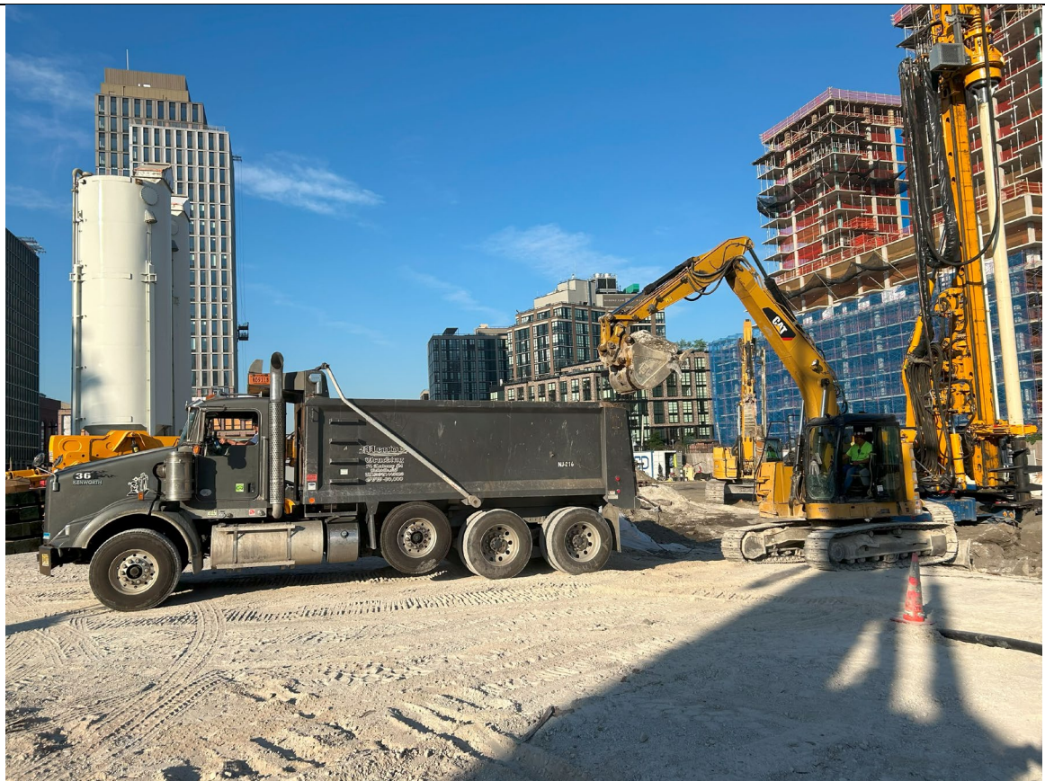
Photo 4 – Representative photo of concrete load out.
