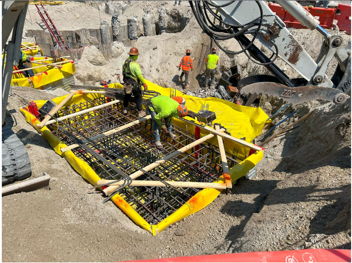
Photo 3 – Representative photo of foundation work and vapor barrier installation.
