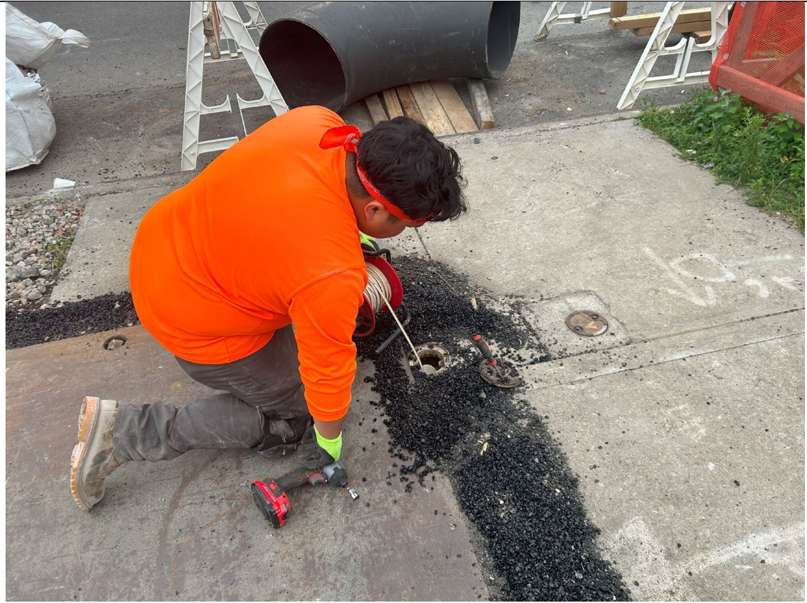
Photo 5 – Representative photo of Sentinel well gauging.
