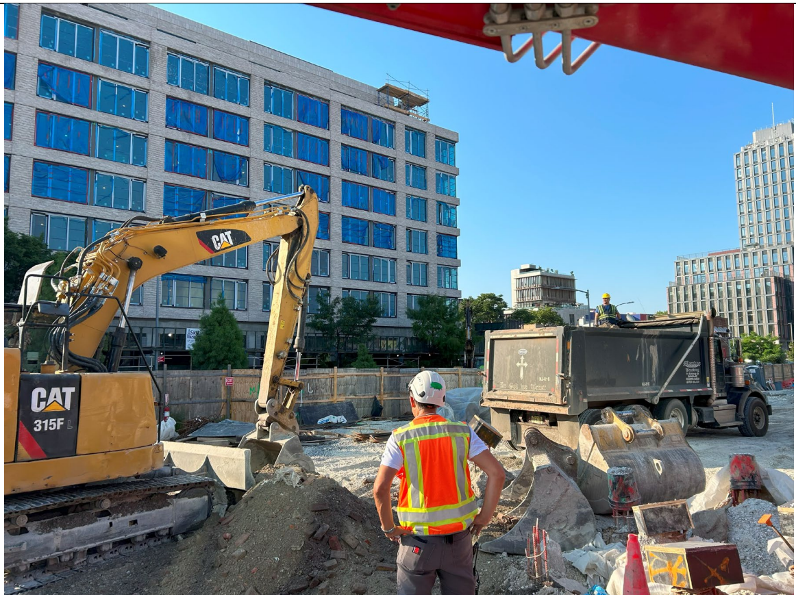
Photo 4 – Representative photo of soil load out.
