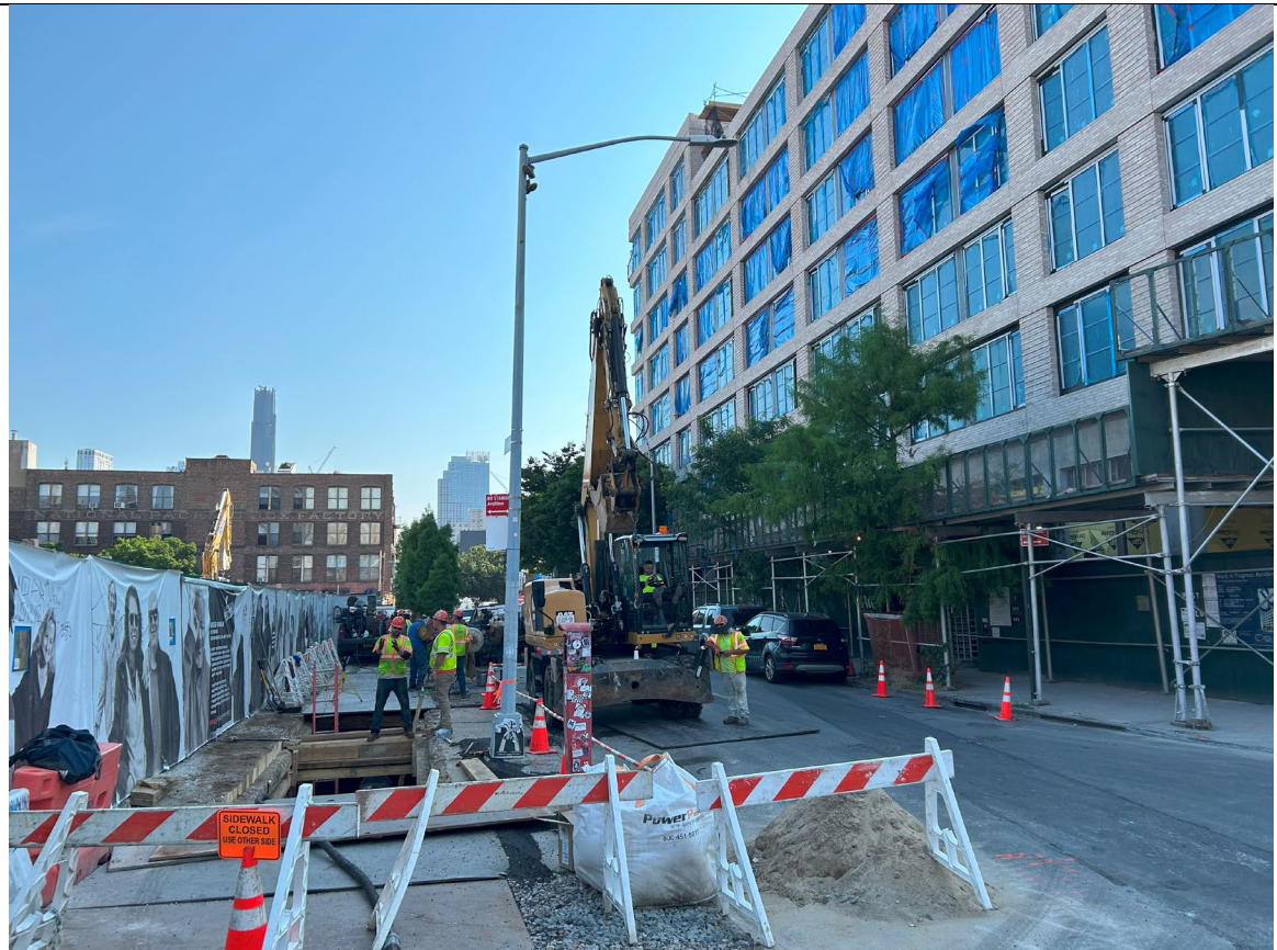
Photo 2 – Representative photo of National Grid gas line work along Nevins Street.
