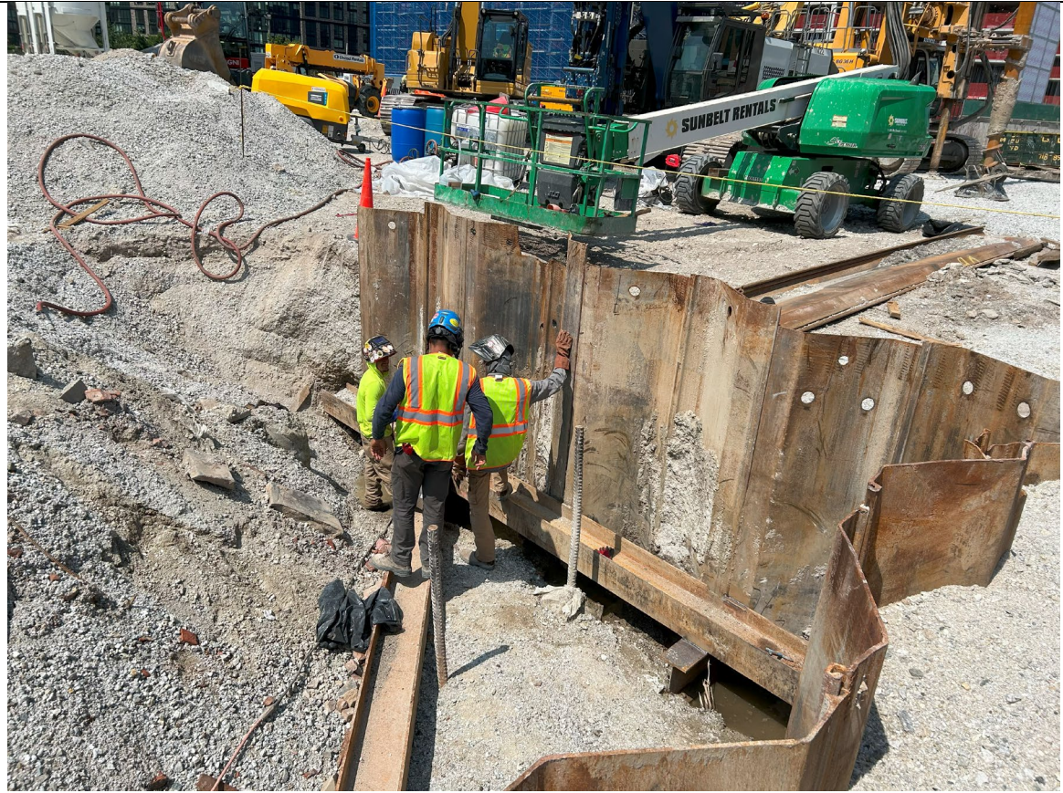
Photo 3 – Representative photo of welding sheeting.
