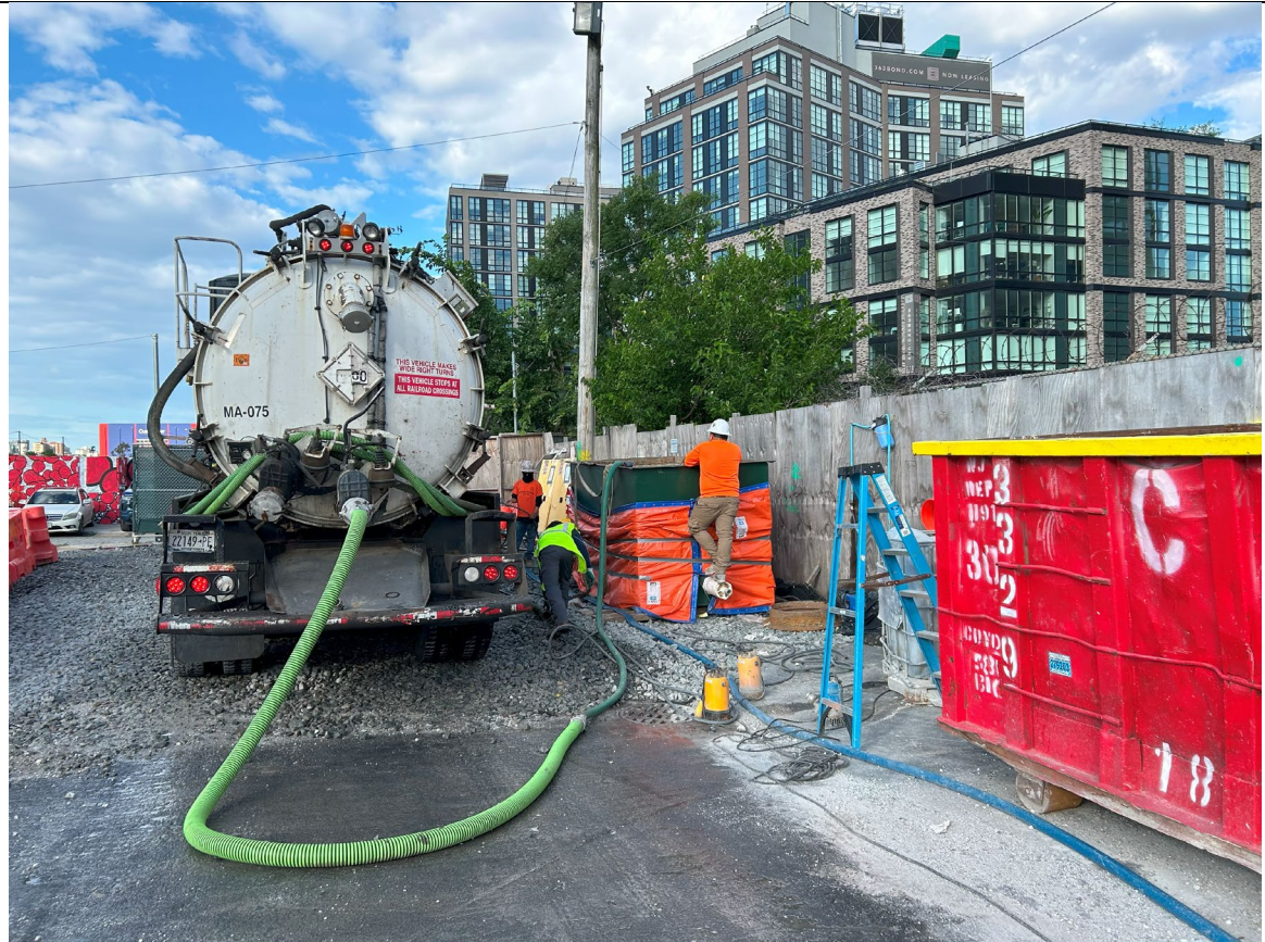
Photo 4 – Representative photo of Triumvirate pumping out truck wash tank.
