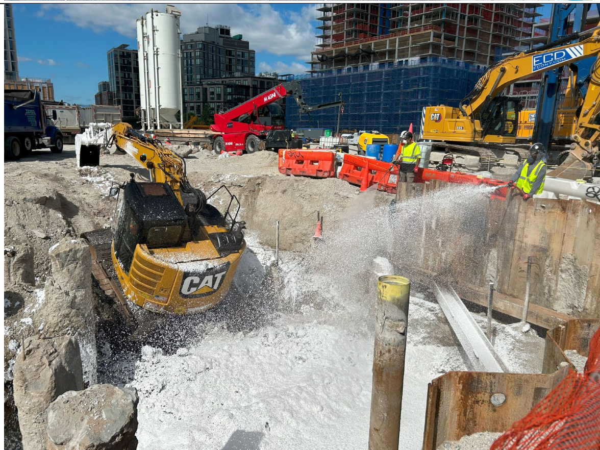
Photo 5 – Representative photo of excavation of Spill 2308807 area material, ATMOS odor suppressant applied to excavation.
