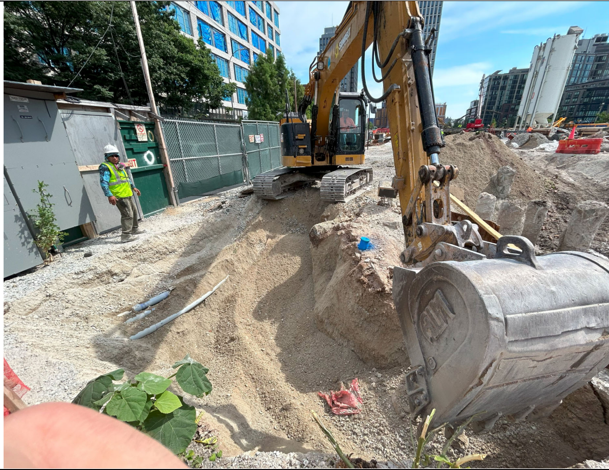
Photo 6 – Representative photo of excavation of EP- 114.
