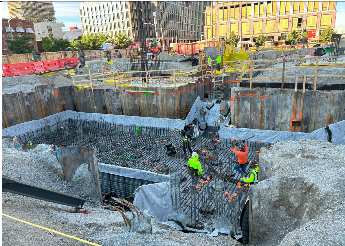
Photo 1 – Representative photo of south building cellar construction.
