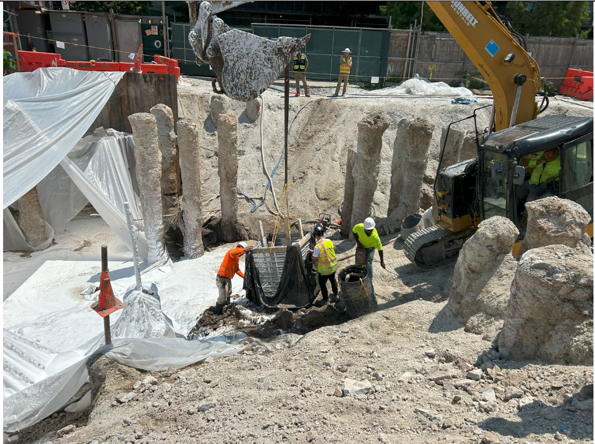
Photo 3 – Representative photo of sump installation in EP- 90.
