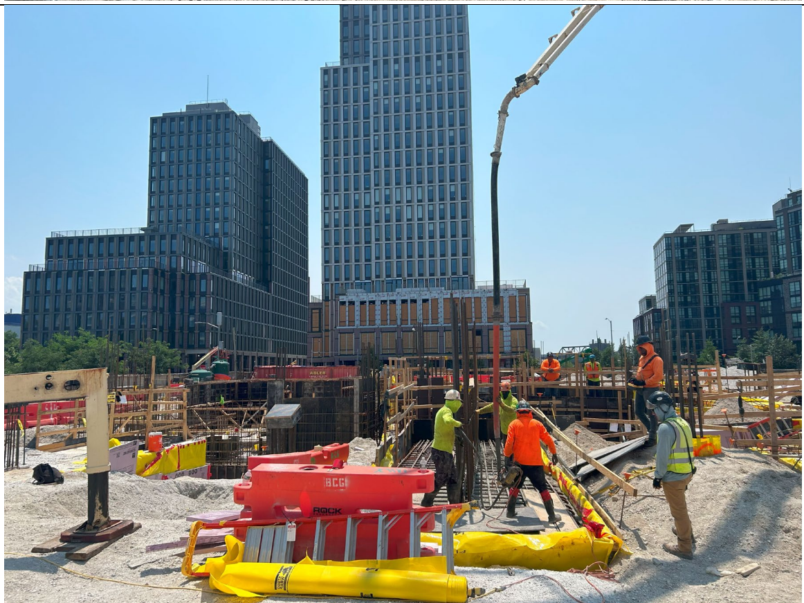
Photo 4 – Representative photo of concrete pour in the south building.
