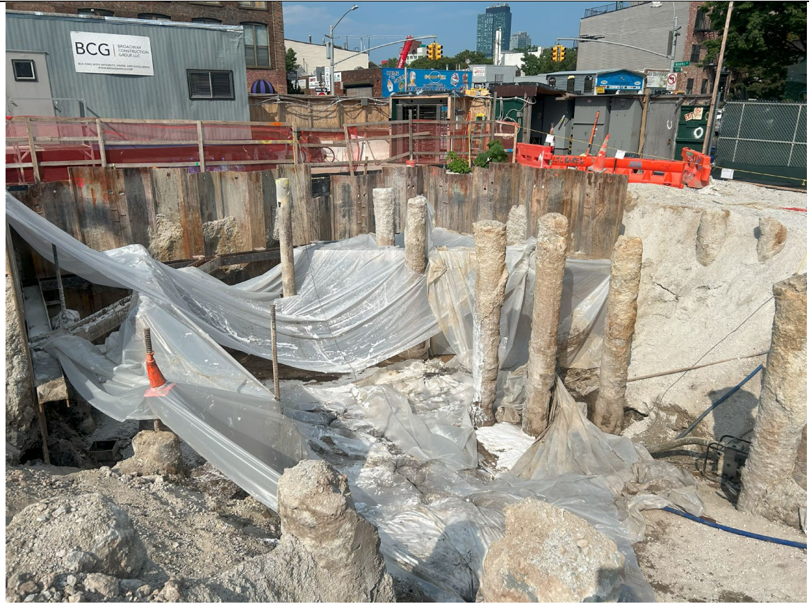
Photo 5 – Representative photo of spill 2308807 area covered with poly at the end of day.
