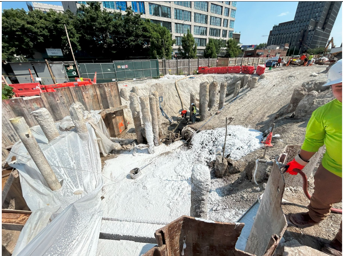
Photo 4 – Representative photo of ATMOS foam being applied to spill area.
