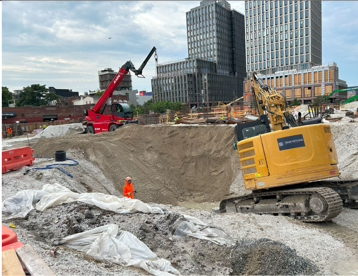
Photo 3 – Representative photo of EP-38 excavation.
