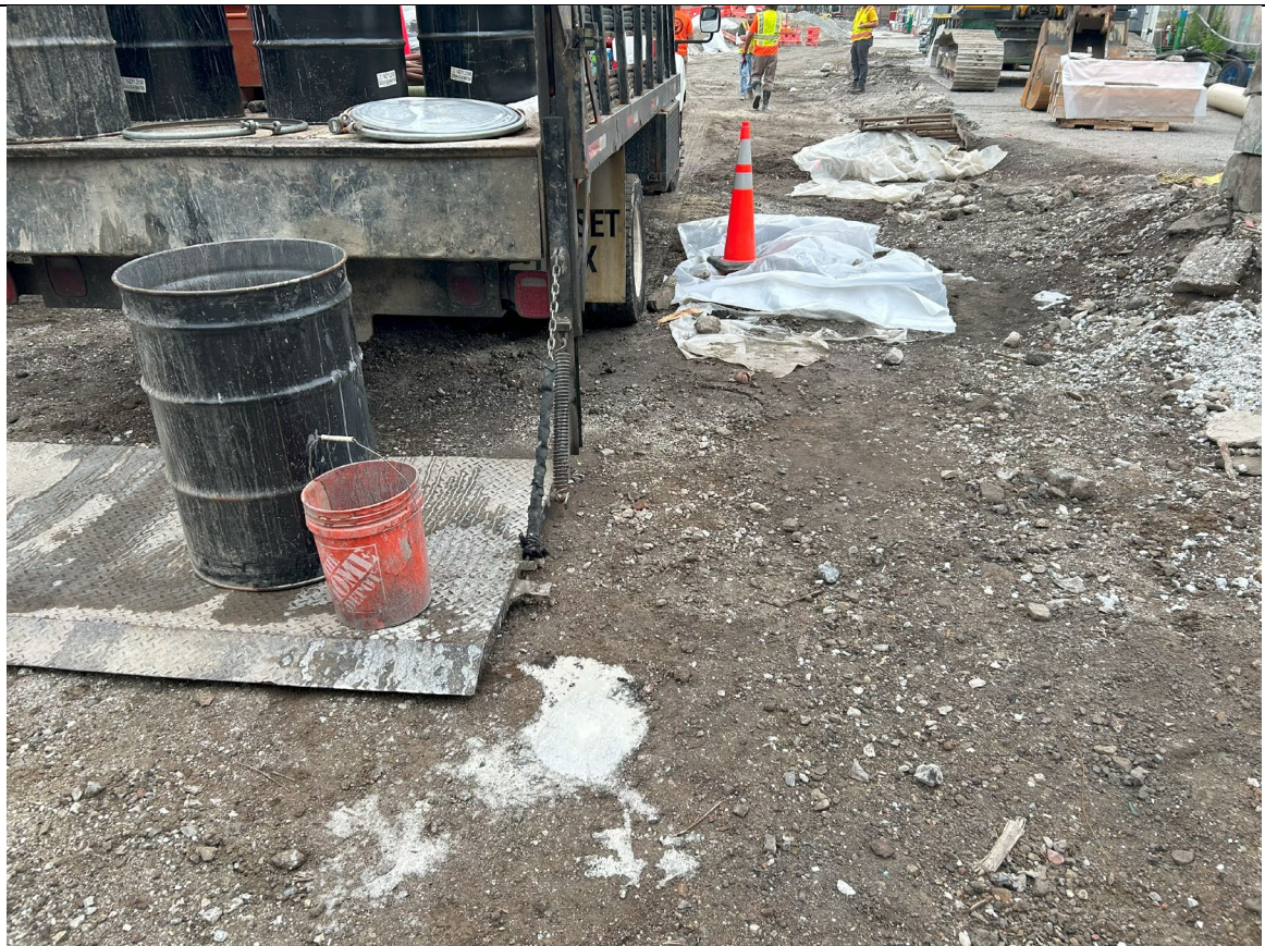
Photo 4 – Representative photo of grouted ISS column boreholes.
