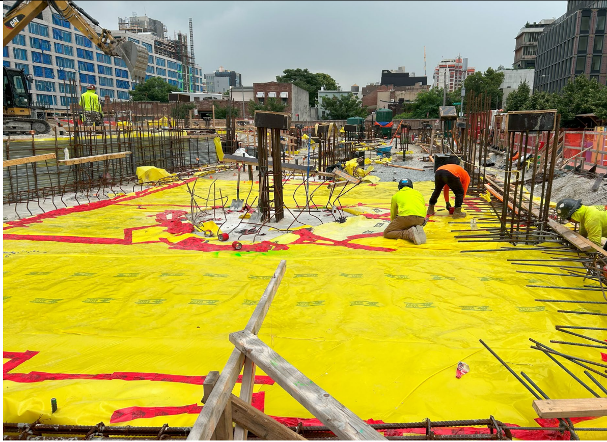
Photo 1 – Representative photo of vapor barrier installation in the south building.
