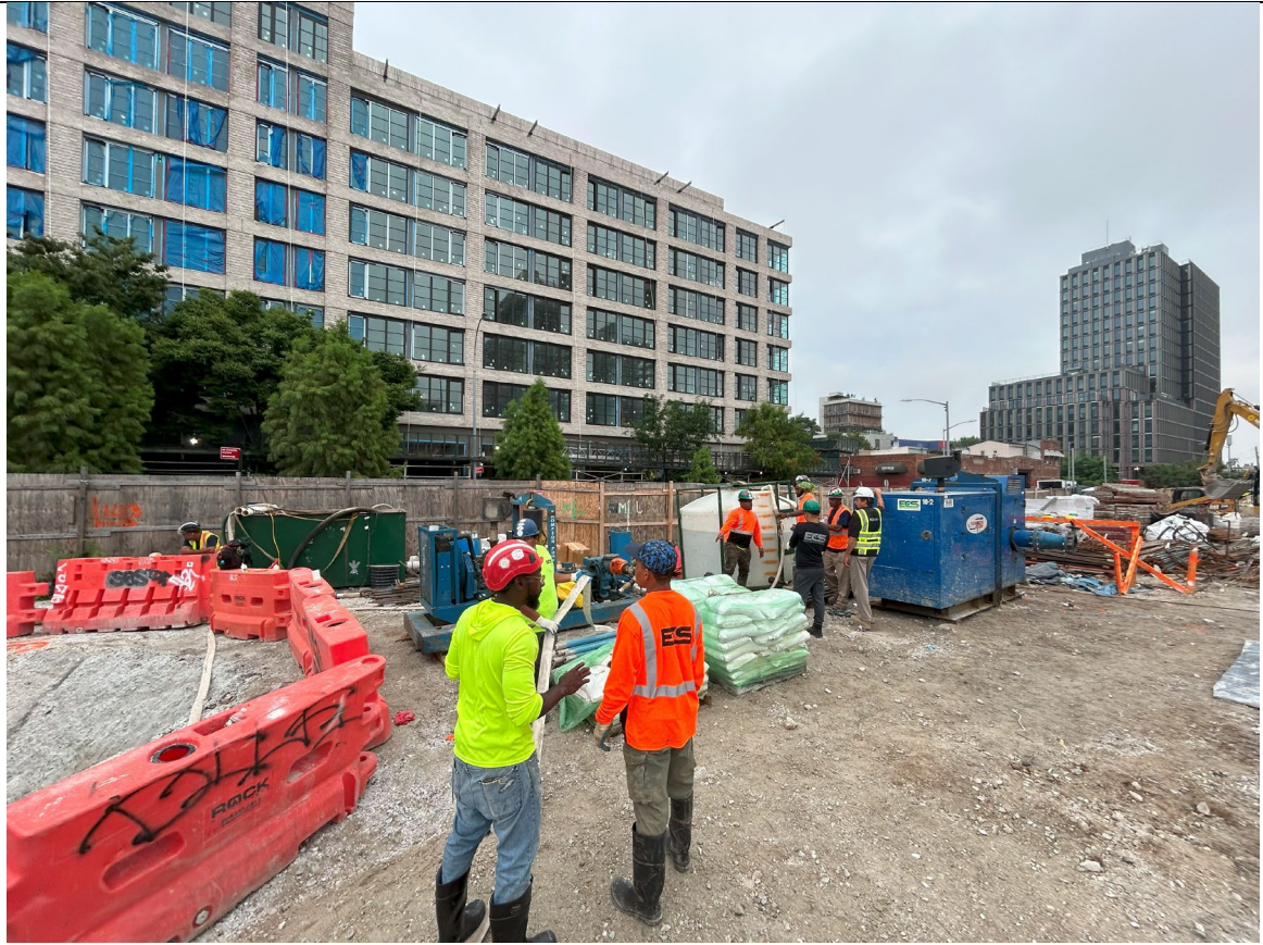
Photo 3 – Representative photo of ECS setting up Well Point pump.
