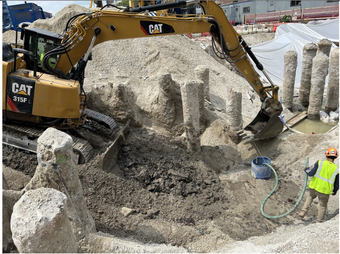
Photo 3 – Representative photo of EP-103 excavation and dewatering sump.
