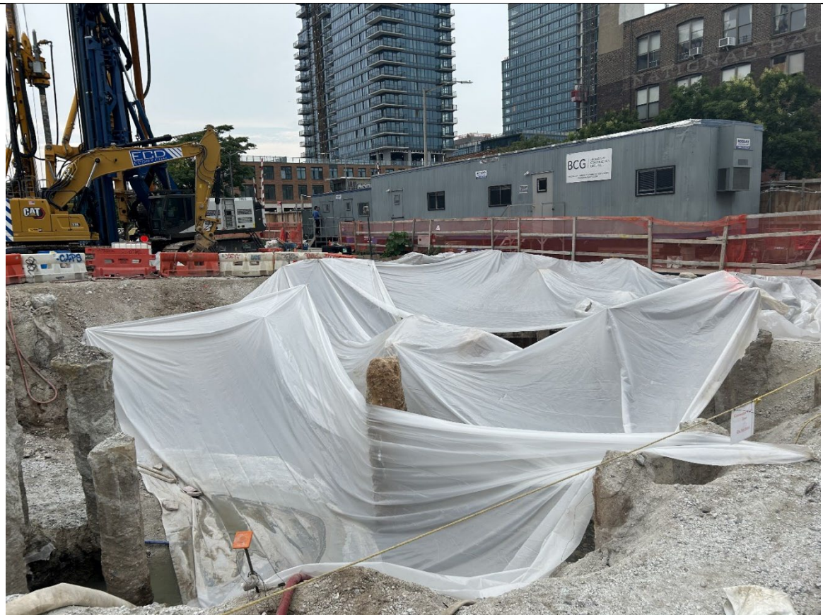
Photo 4 – Representative photo Spill 2308807 covered with poly by the end of day.
