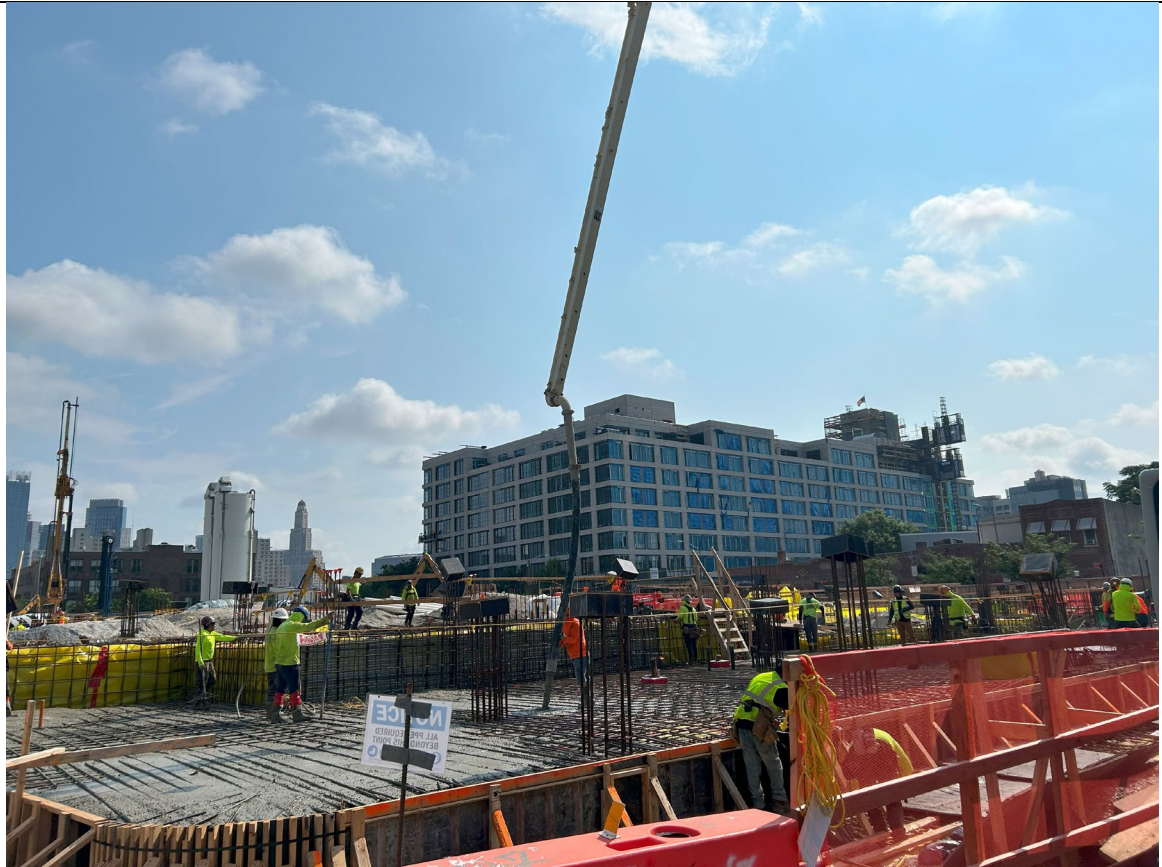
Photo 3 – Representative photo of concrete pour in the south building.
