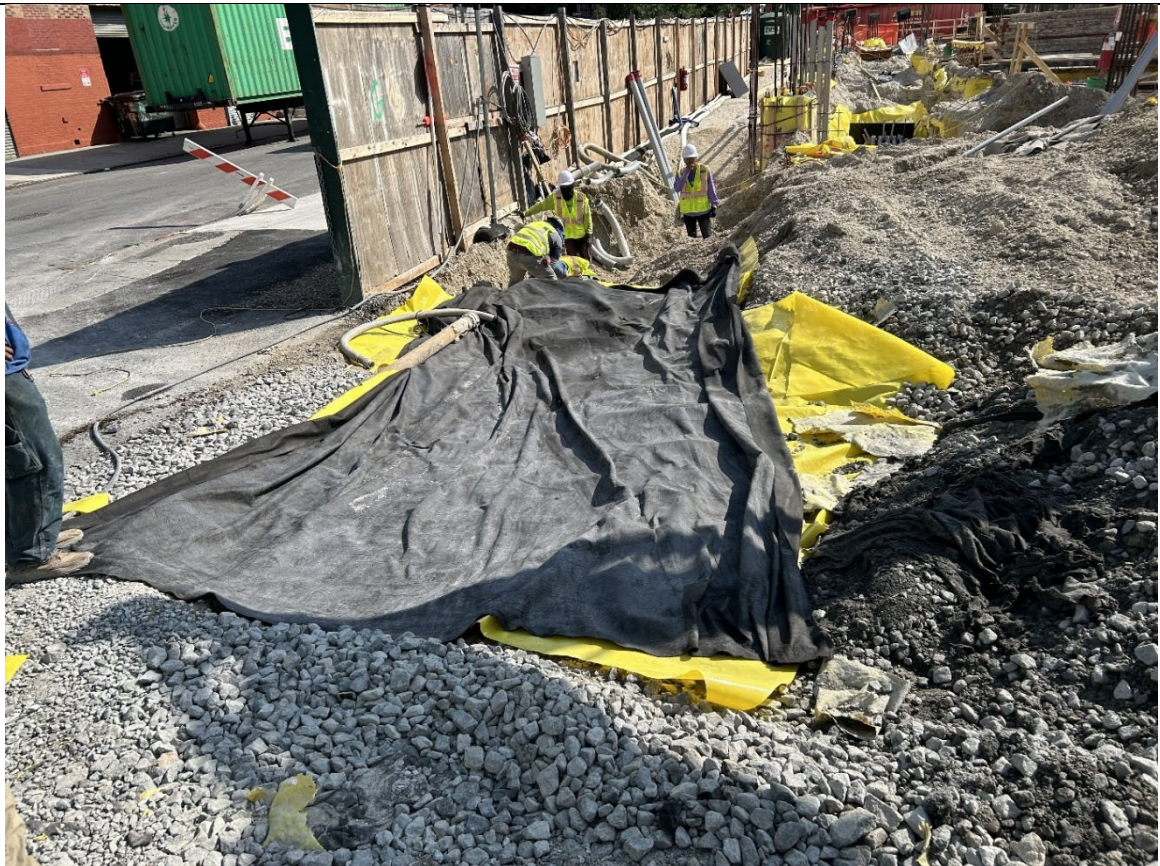
Photo 2 – Representative photo of patching of truck wash pad lining.
