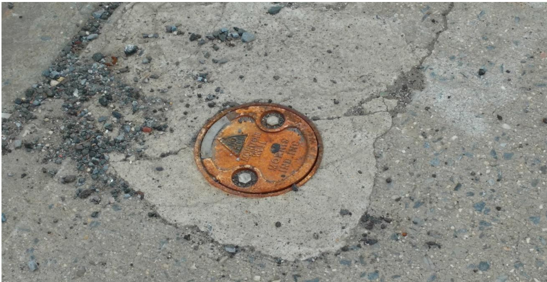
Photo 14: View of a groundwater monitoring well installed in the Pennsylvania Avenue sidewalk east of the eastern adjoining property.
