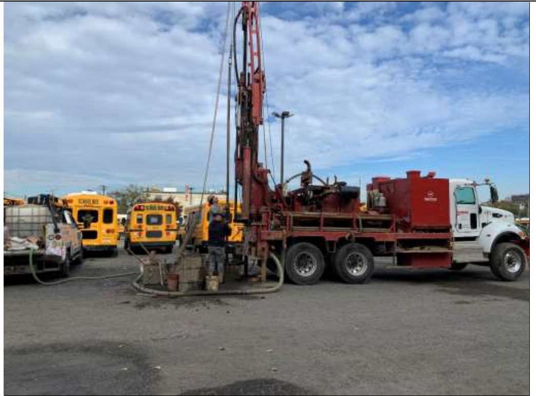
Photo 1 – Craig drilling at B-15, facing west.
