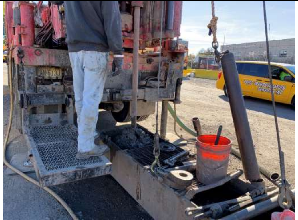
Photo 1 – Craig drilling boring B-4, facing southeast.
