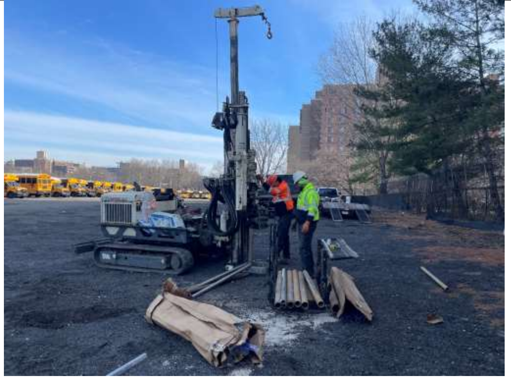
Photo 1 – AARCO drilling at LSB-40, facing east.
