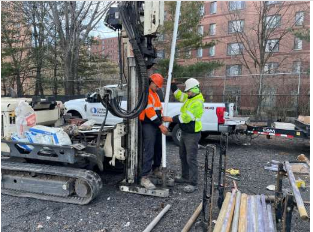
Photo 2 – AARCO installing LMW-22 at LSB-41, facing south.
