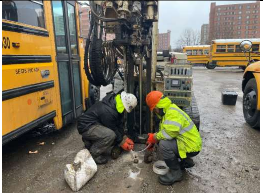
Photo 1 – AARCO installing LSV-10, facing south.
