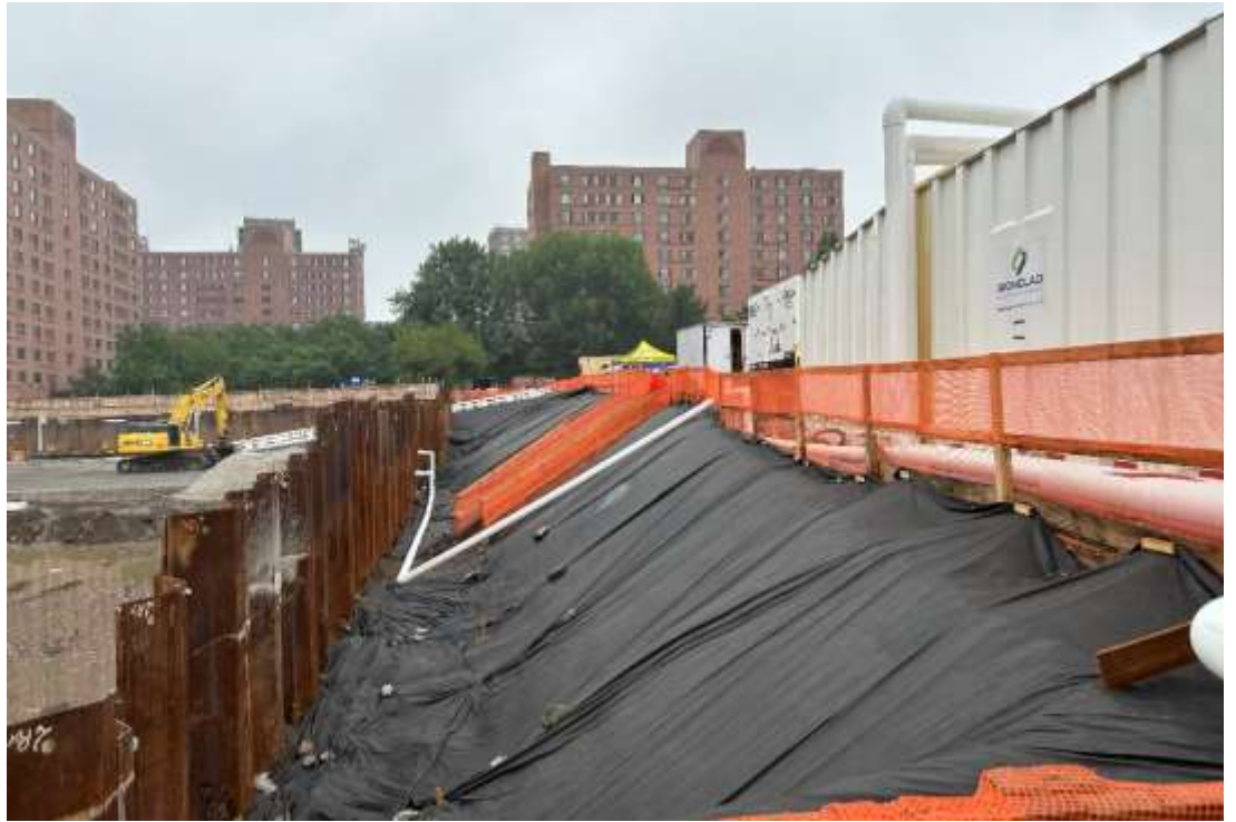
Photo 3 – View of filter fabric above exposed soil in the northeastern portion of the Site, facing south.
