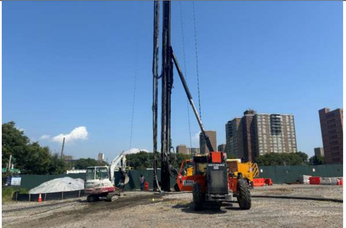
Photo 1 – Morris-Shea installing foundation test piles in the northern portion of the Site, facing east.
