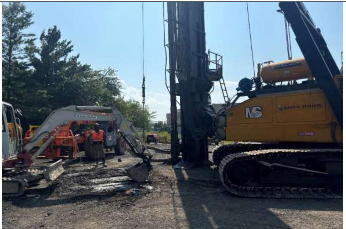
Photo 2 – Morris-Shea installing foundation test piles in the southern portion of the Site, facing southwest.
