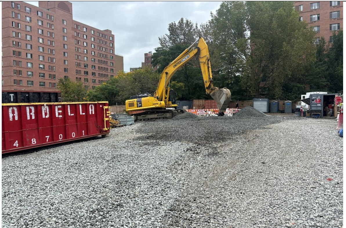
Photo 2 – United spreading stone over the logistical zone, facing south.
