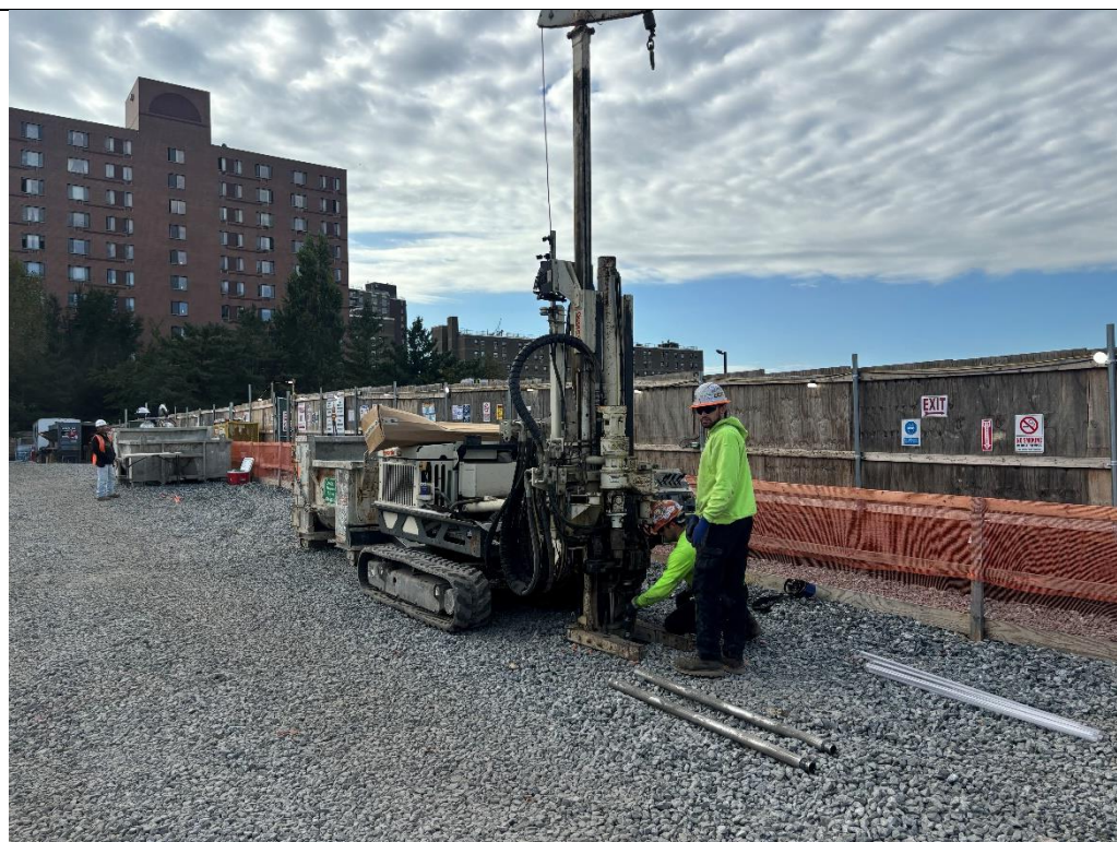
Photo 3 – AARCO advancing soil boring LSB204 in the central portion of the Site within the logistical zone, facing southwest.
