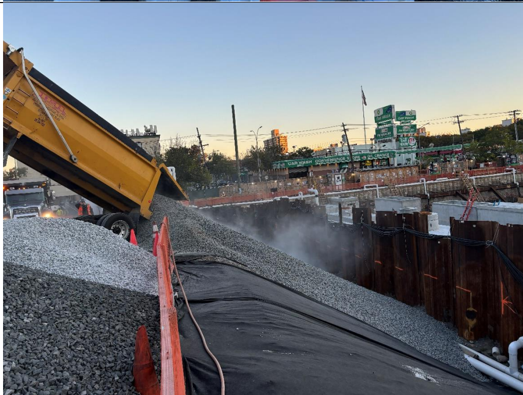
Photo 4 – United importing 1.5-inch stone and backfilling in the northeastern portion of the Site.
