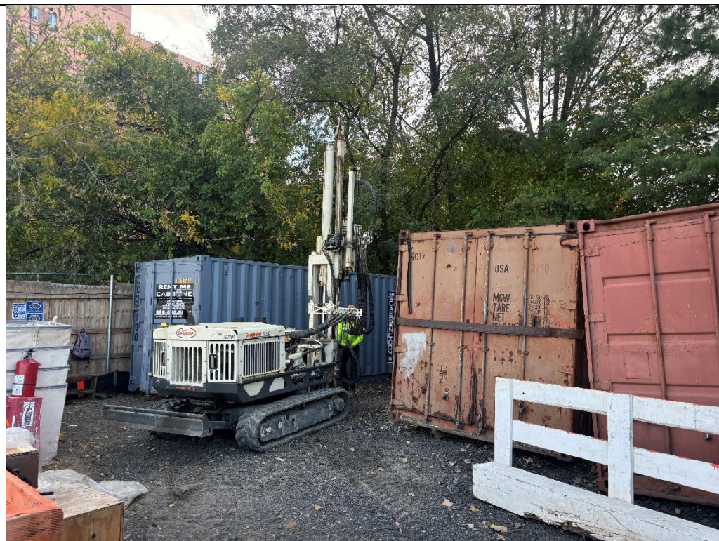
Photo 3 – AARCO advancing soil boring LSB42_2_N5 in the southern portion of the Site, facing southeast.
