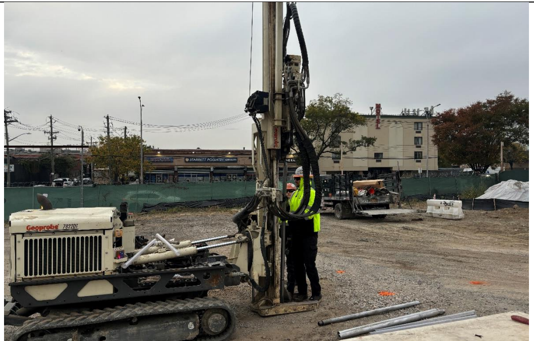
Photo 1 – AARCO advancing soil boring LSB133_2_W5 in the northern portion of the Site, facing north.
