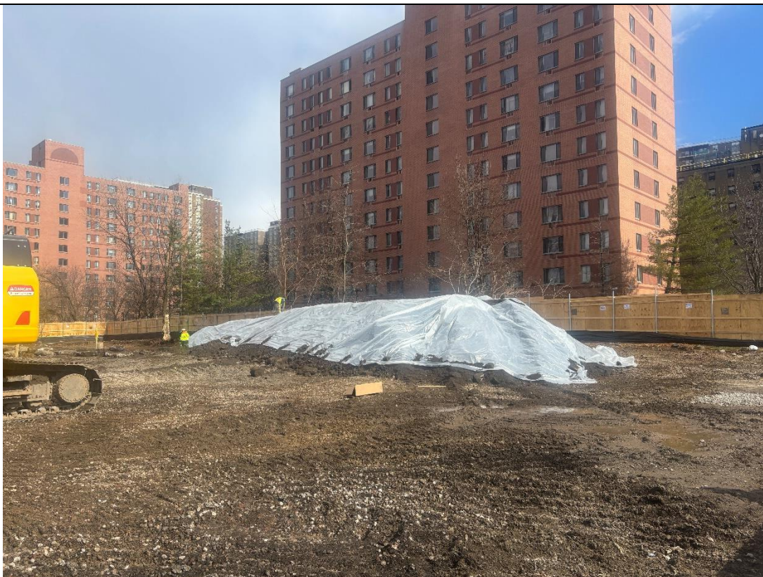
Photo 4 – View of stockpile ST-1 covered with polyethylene sheeting, staged in the southern portion of the Site for future off-Site disposal, facing southeast.
