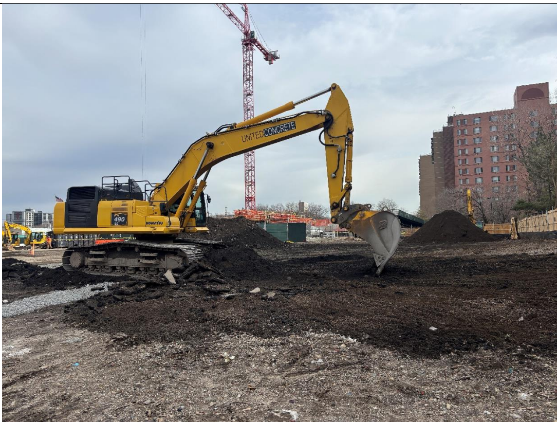
Photo 3 – United removing asphalt pavement in the southeastern portion of the Site for future off-Site disposal, facing east.
