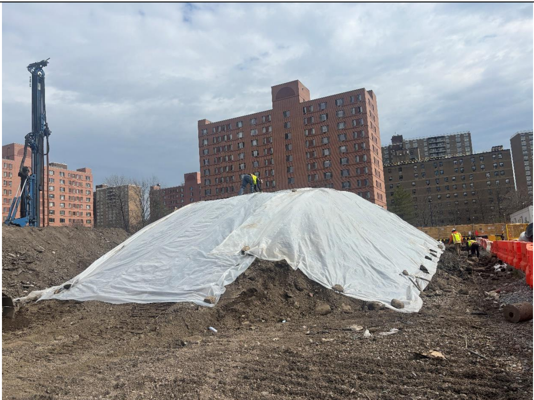
Photo 4 – United covering stockpile ST-1 at the end of the day, facing south.
