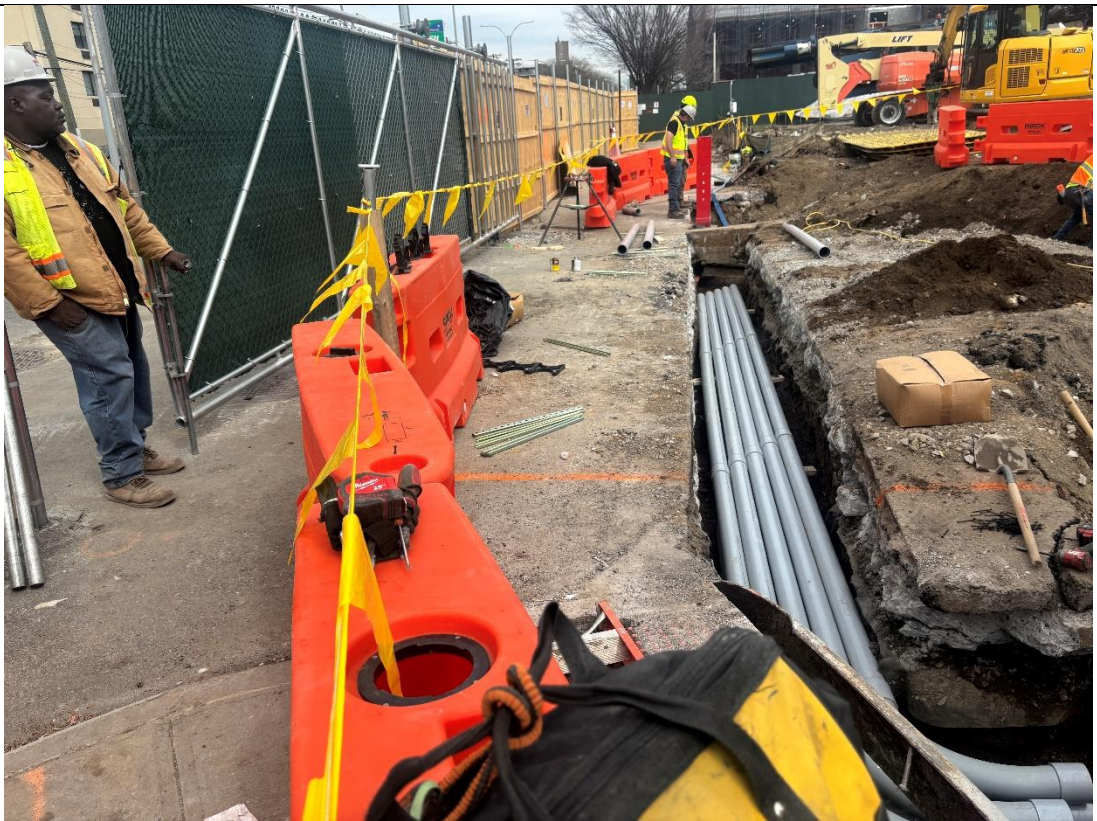
Photo 3 – United relocating the temporary electric lines to the sidewalk north of the BCP Site boundary, facing east.
